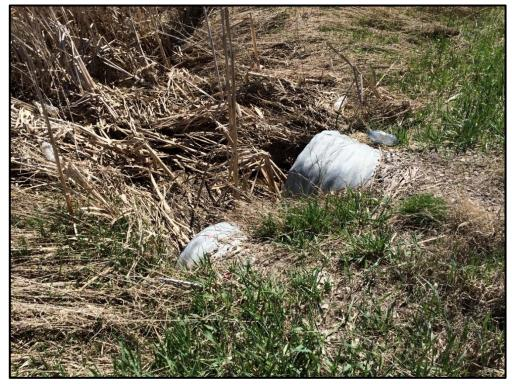
Photo 41: Crossing RS1, downstream ROW, twin CSP culverts.
