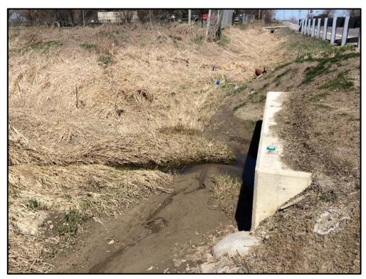
Photo 9: Upstream end of Crossing RB2. Note ditch drainage outletting from the west of the watercourse.
