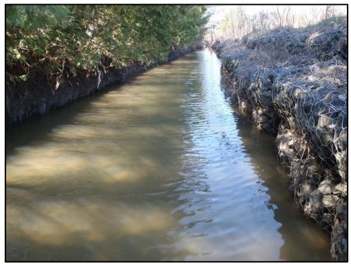
Photo 13: CTA, facing upstream (north). Note gabion baskets and channelization.
