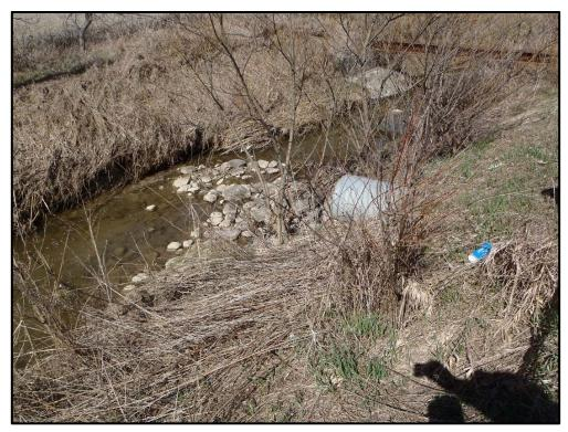
Photo 22: CTA, Reach 5. Another culvert outlets to the stream from the east. Culvert conveys flows from dry agricultural drainage ditch under the road.
