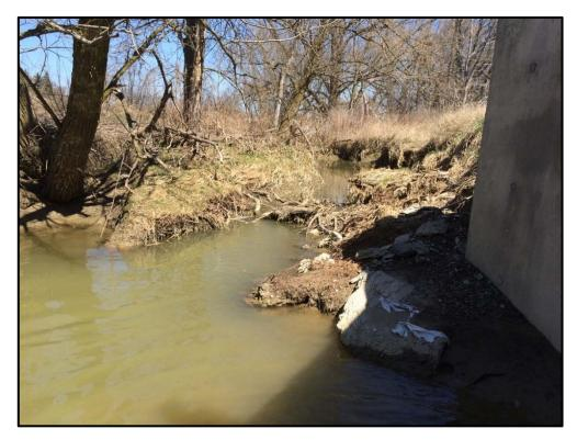
Photo 38: Crossing CT5, ROW to 20 m upstream area. Note failing bank on south bank of stream adjacent to roadway.
