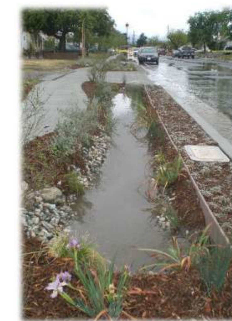
Example of roadside LID (Bioswale)
