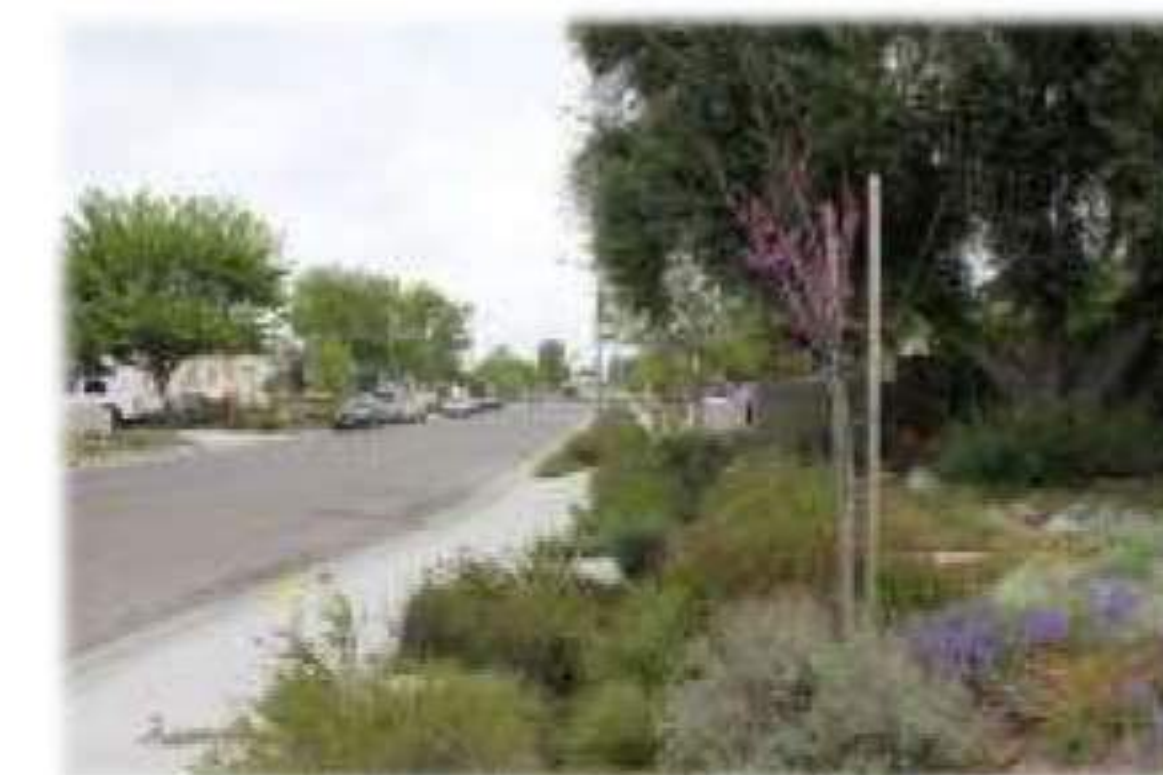
Example of roadside LID (Rain Garden)
