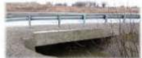
Clarkway Drive over Clarkway Tributary
