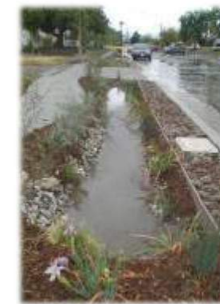
Example of roadside LID (Bioswale)
