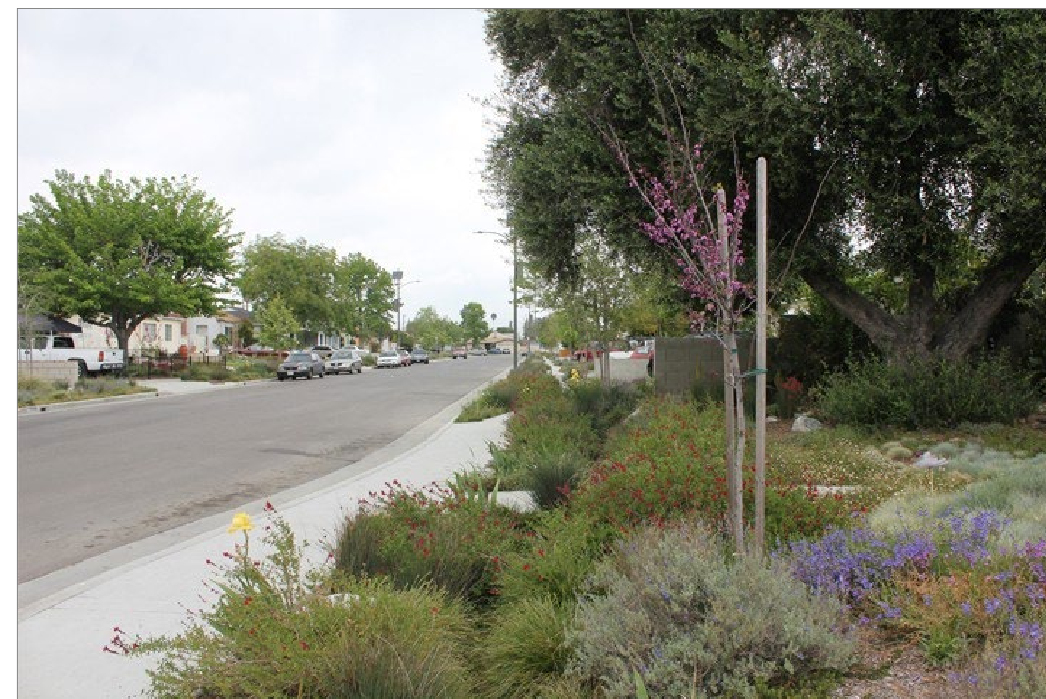
Example of roadside LID (Rain Garden)
