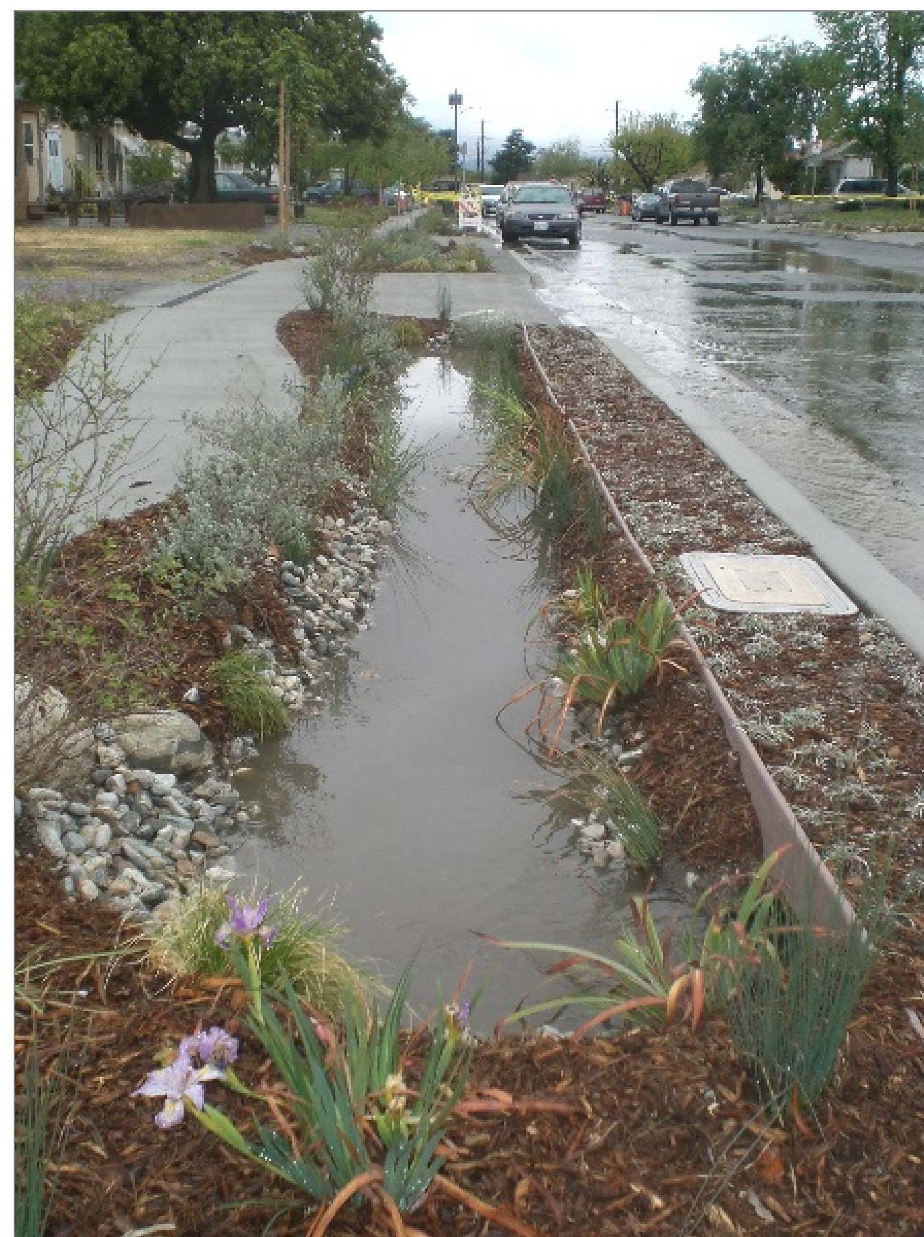
Example of roadside LID (Bioswale)
