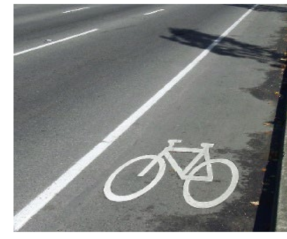
On-street bike lanes Cyclists travel on-street adjacent to traffic lanes
