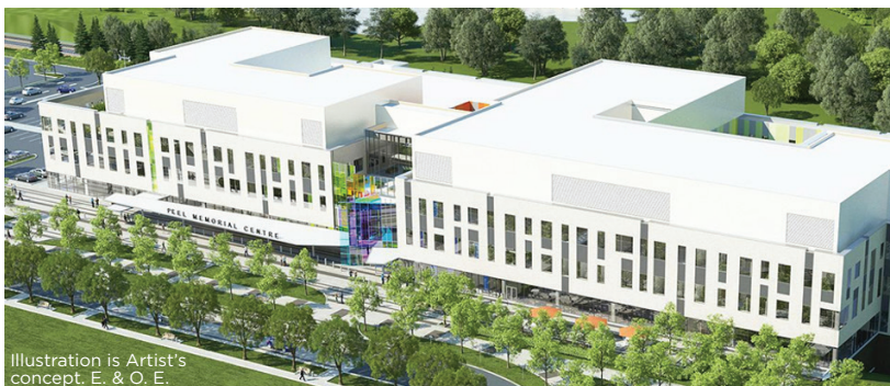
Peel Memorial Phase II expansion
