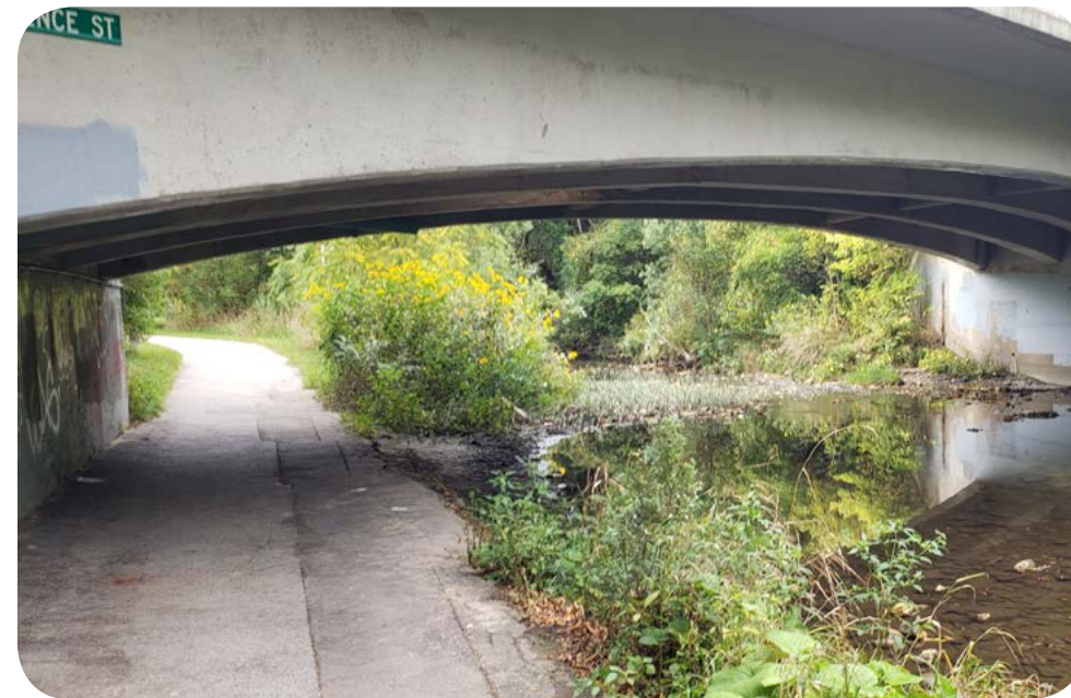
Trail Beneath Clarence Street Bridge
