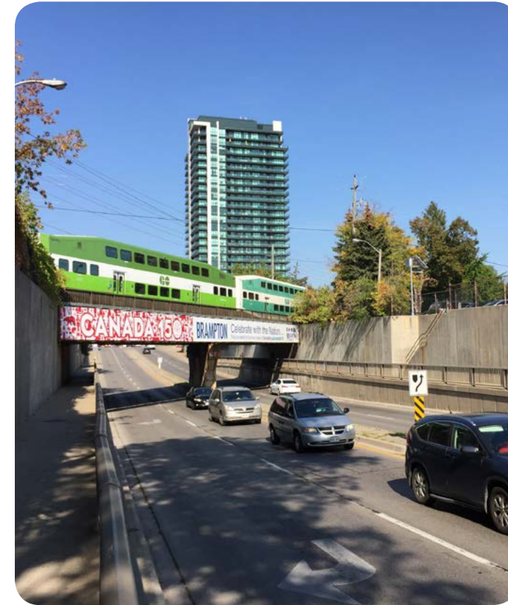
Queen Street Underpass
