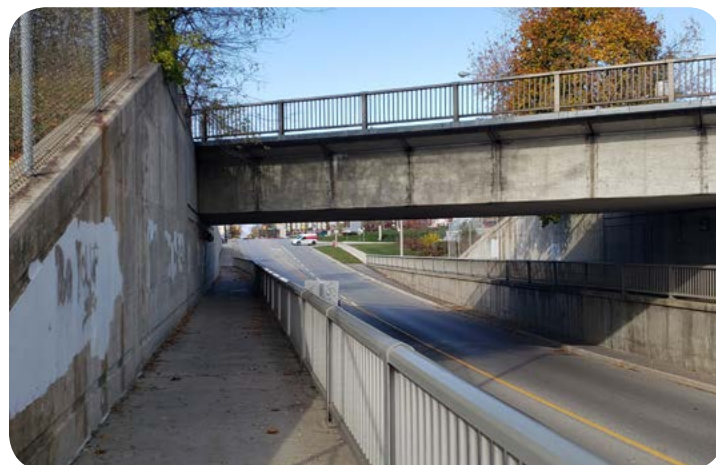
Centre Street Rail Underpass
