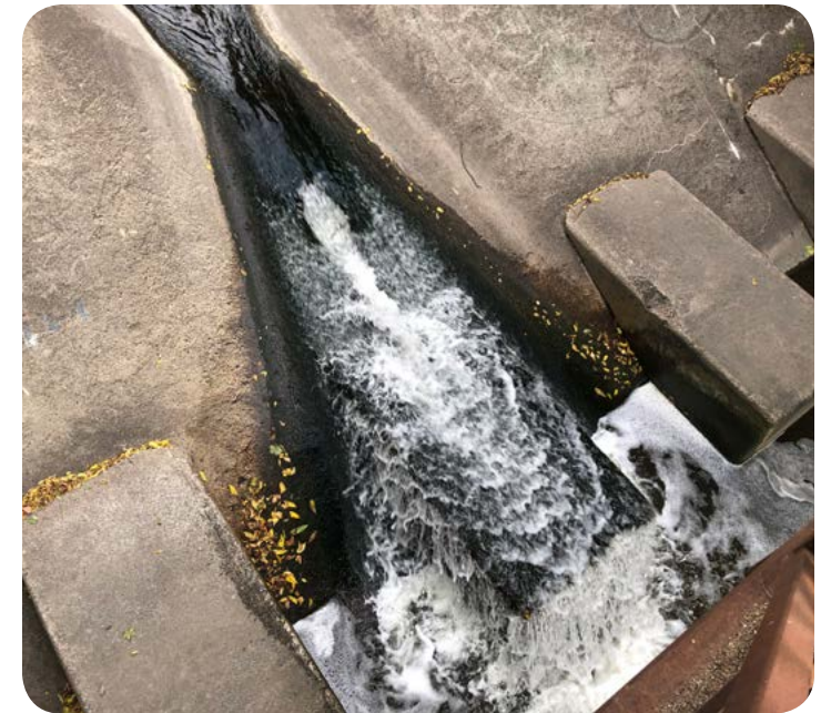
Etobicoke Creek Bypass Channel Weir at CN Bridge
