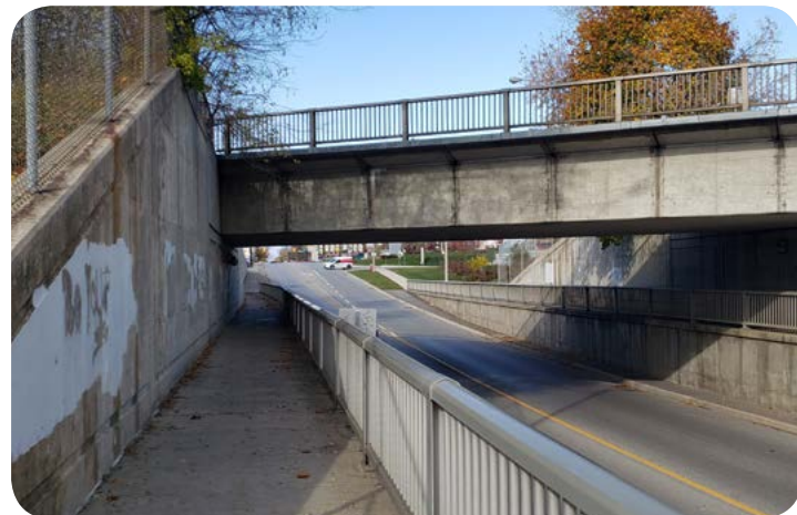
Centre Street Rail Underpass
