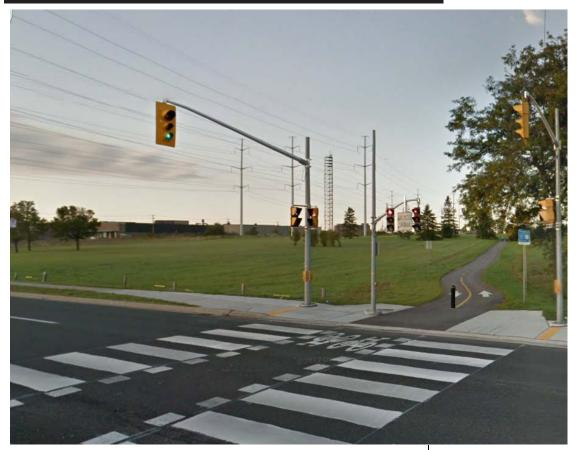
This photo is an example of the types of pavement markings that may be suitable at a signalized trail crossing where there is a lot of motor vehicle traffic.
