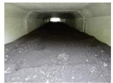
Wildlife crossing structure (concrete culvert)
