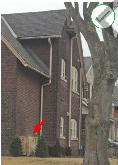
Figure 45. An example of screening where a heat pump would otherwise be visible on a corner lot. (Source: ERA)
