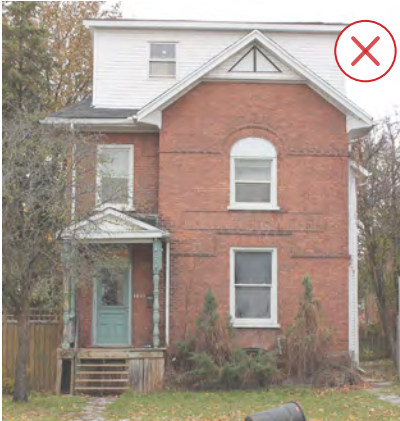
Figure 55. This rooftop addition is not in keeping with the character of the house. It changes the basic shape of the building and uses a material palette that is not complementary to the rest of the building. The window in the addition does not fit with the size and location of other windows. (Source: ERA)
