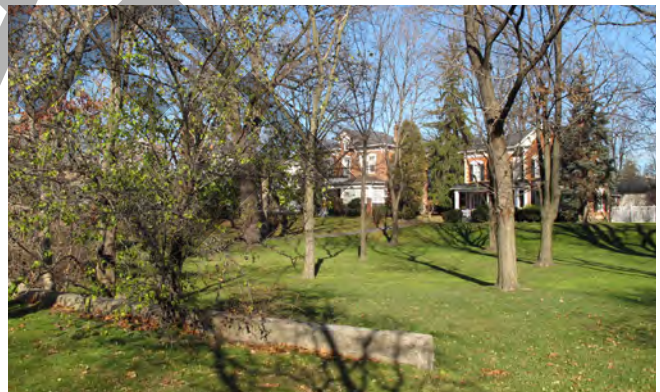
Figure 94. Remaining retaining wall. (Source: ERA)
