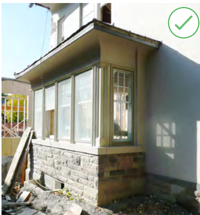
Figure 52. This small addition was designed in a way that adds to the character of the house. It reflects the existing style and material palette. For example, the stone base references the existing stone foundation. (Source: ERA)
