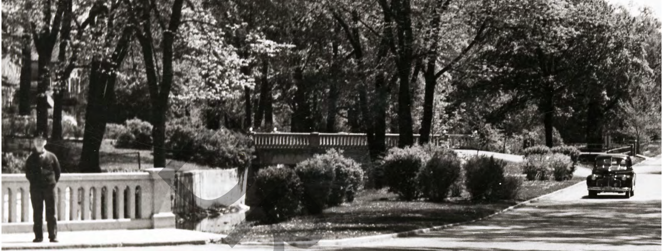
Figure 92. Driveway bridge from street to 58 Main Street South. (Source: PAMA)
