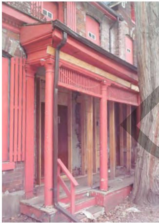
Figure 42. Existing condition. (Source: ERA)
