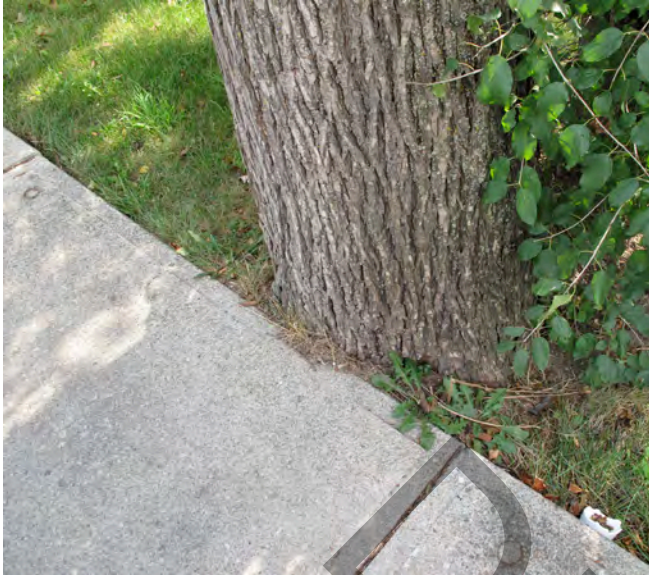
Figure 85. Widening of the roadway has encroached on this tree's root system. (Source: ERA)
