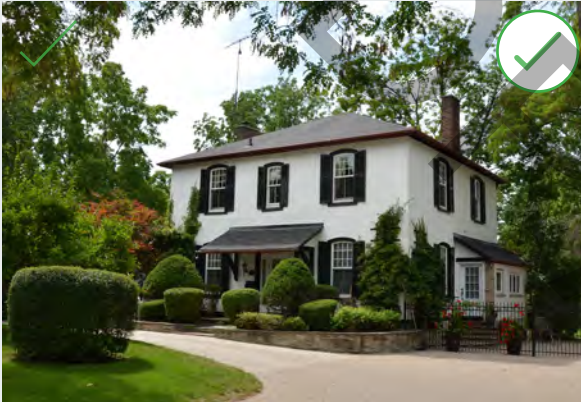
Figure 19. Historic use of traditional lime-based stucco or render in the District at 93 Main Street South. (Source: ERA)
