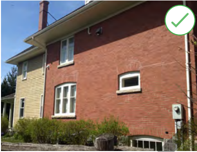
Figure 54. This side addition fits well with the main building. It is set back from the side elevation, its windows are in proportion to the original windows, and it is clad in a material that complements the original brick. (Source: City of Brampton)
