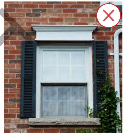
Figure 37. This photo shows storm shutters that are not appropriately sized for the window (Source: City of Brampton)
