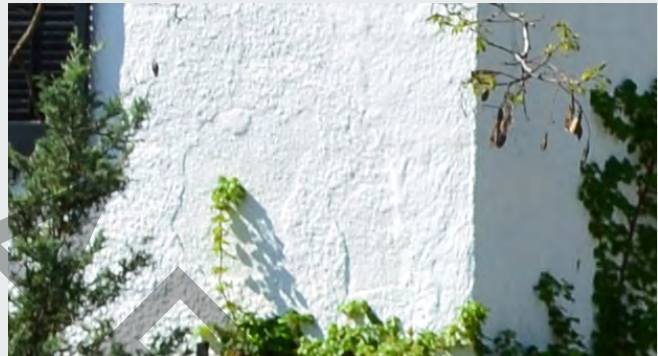
Figure 20. Close-up of 93 Main Street South traditional stucco work to show rich, irregular texture. (Source: ERA)
