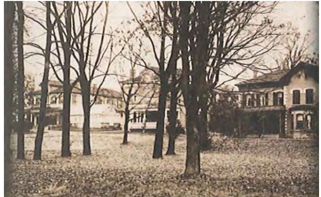
Figure 78. Early photograph of 52, 56, 58 Main Street South showing the tree canopy on deep lots is vital to the park-like character of the District. Date unknown. (Source: City of Brampton)
