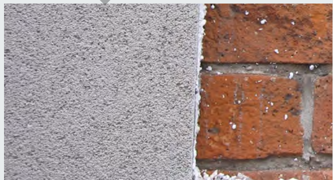
Figure 22. Use of synthetic cladding over masonry at 300 King, Toronto. (Source: ERA)
