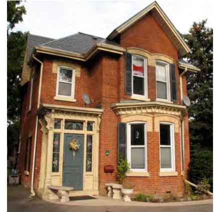
Figure 39. The door and entryway details can be defining features of a building. These have been maintained on this house. (Source: ERA)
