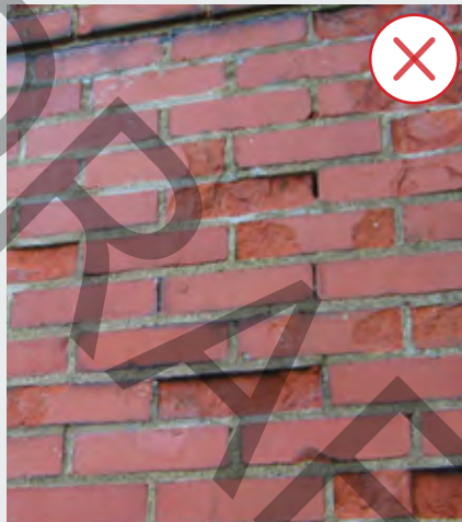
Figure 18. Left: Spalling as a result of improper maintenance. Right: Regular maintenance, such as re-pointing brick and/or stone masonry, is encouraged. (Source: ERA)
