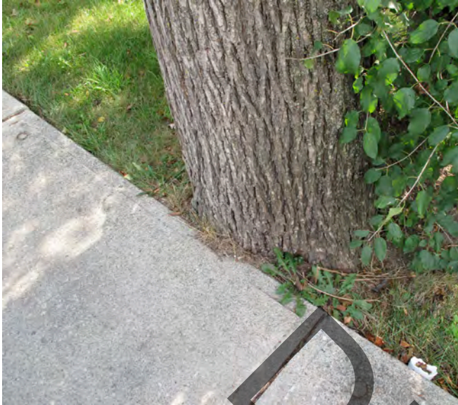
Figure 85. Widening of the roadway has encroached on this tree's root system. (Source: ERA)
