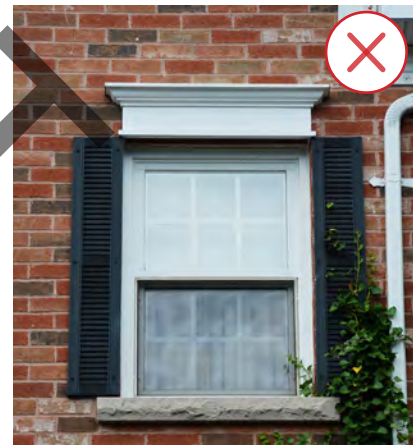
Figure 38. This photo shows storm shutters fixed in place. (Source: City of Brampton)
