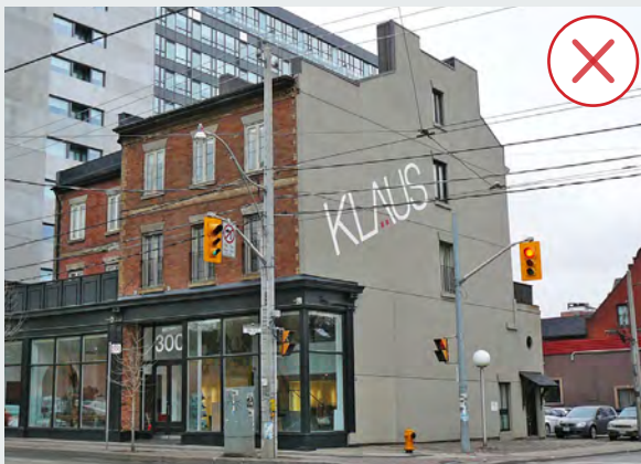
Figure 22. Detail and cut-away sample of the exterior wall showing the uniform texture of the synthetic stucco and the damaging to the masonry underneath. (Source: ERA)
