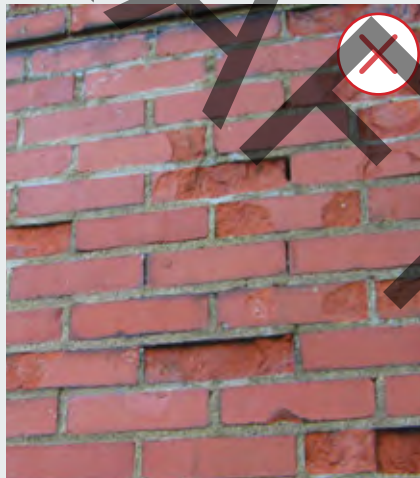
Figure 19. Left: Spalling as a result of improper maintenance. Right: Regular maintenance, such as re-pointing brick and/or stone masonry, is encouraged. (Source: ERA)
