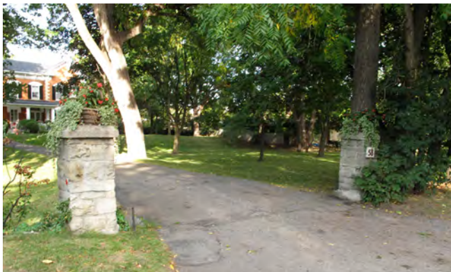
Figure 93. Remaining bridge posts. (Source: ERA)
