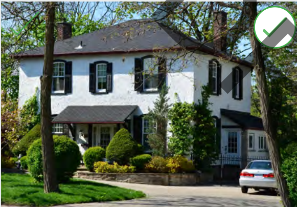
Figure 20. Historic use of traditional lime-based stucco or render in the District at 93 Main Street South. (Source: ERA)
