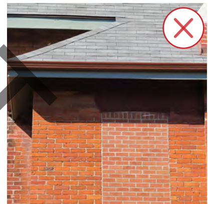
Figure 35. This photos shows a window opening bricked in. (Source: ERA)
