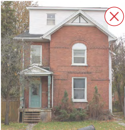
Figure 56. This rooftop addition is not in keeping with the character of the house. It changes the basic shape of building and uses a material palette that is not complimentary to the rest of the building. The window in the addition does not fit with the size and location of other windows. (Source: ERA)
