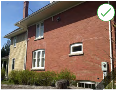
Figure 55. This side addition fits well with the main building. It is set back from the side elevation, its windows are in proportion to the original windows, and it is clad in a material that compliments the original brick. (Source: City of Brampton)
