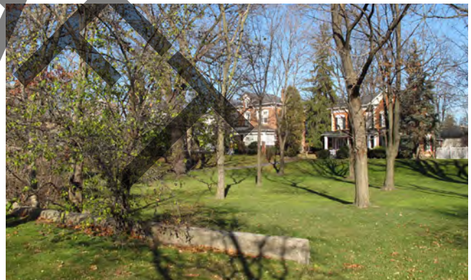
Figure 94. Remaining retaining wall. (Source: ERA)
