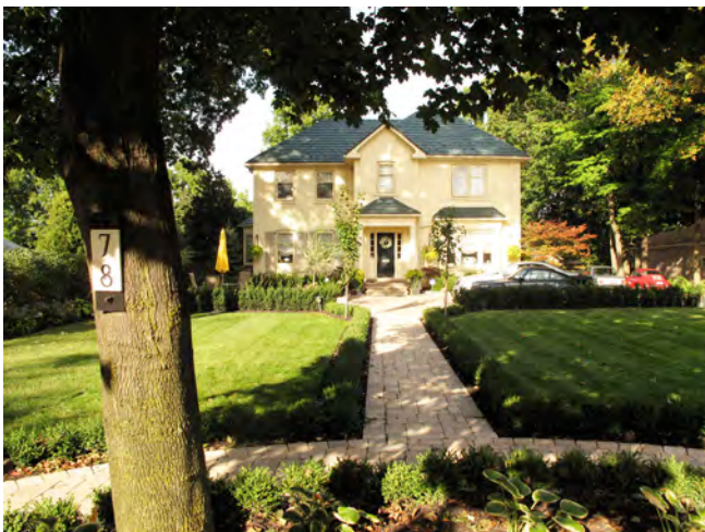
Figure 59. 78 Main Street South is sited perpendicular to Main Street. (Source: ERA)
