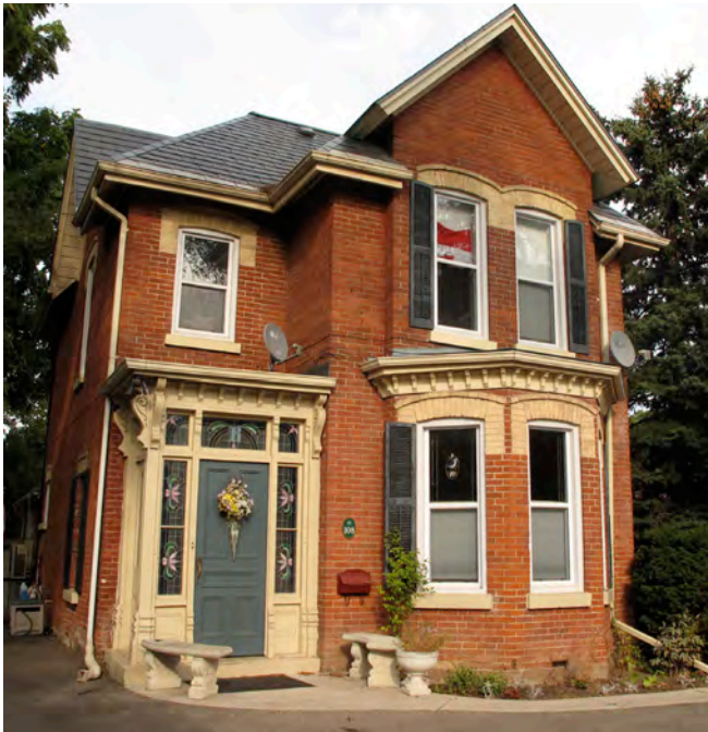
Figure 40. The door and entryway details can be defining features of a building. These have been maintained on this house. (Source: ERA)
