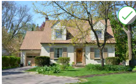
Figure 51. This garage addition uses complimentary materials and building form to maintain the character of the house. (Source: City of Brampton)
