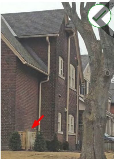
Figure 46. An example of screening where a heat pump would otherwise be visible on a corner lot. (Source: ERA)
