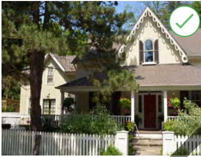
Figure 52. The rear addition on the left of the photograph uses complimentary materials and a similar roof shape to conserve character of the house. (Source: City of Brampton)
