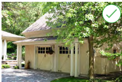
Figure 50. This detached garage addition is set back from the main façade to help maintain the massing and profile of the main building. (Source: City of Brampton)
