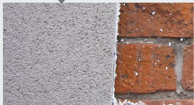
Figure 23. Use of synthetic cladding over masonry at 300 King, Toronto. (Source: ERA)
