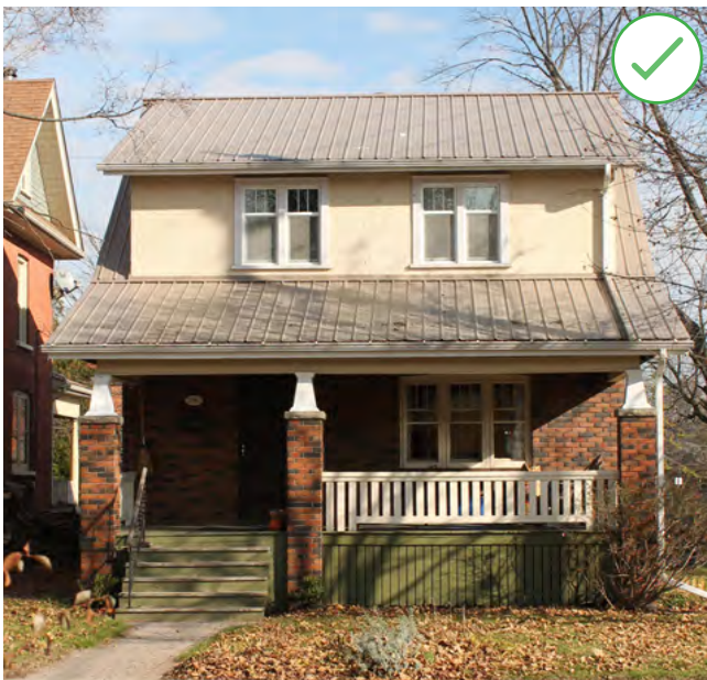
Figure 16. Stucco cladding in this example has been maintained on the dormer. (Source: ERA)
