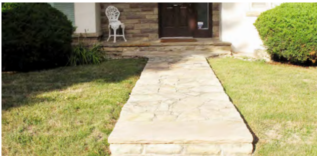
Figure 77. Stone pavers at 68 Main Street South provide a texture to the landscape design. (Source: ERA)
