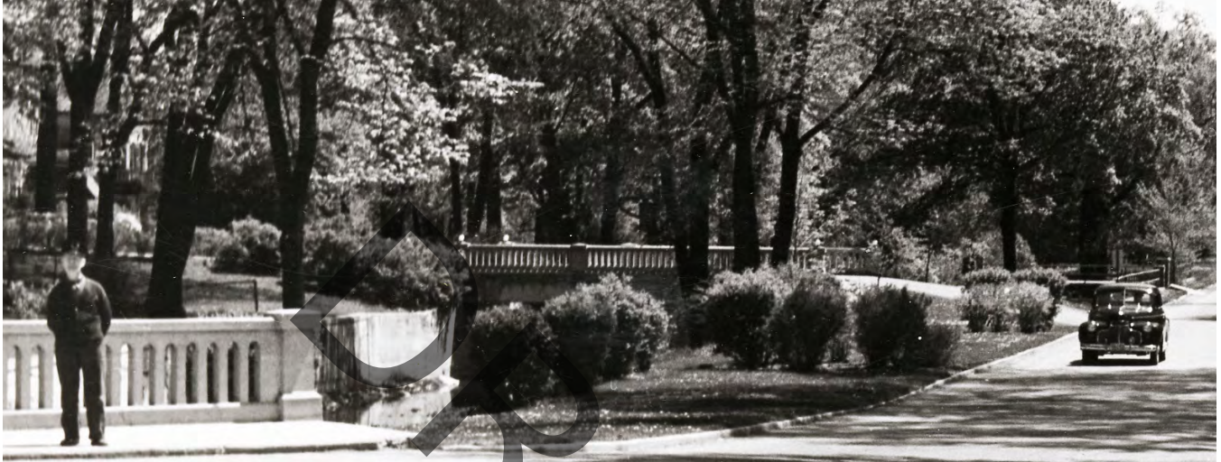
Figure 92. Driveway bridge from street to 58 Main Street South. (Source: City of Brampton)
