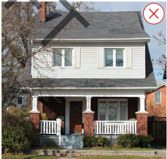
Figure 17. On this house inappropriate siding detracts from the character of a building. (Source: ERA)
