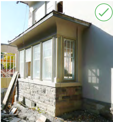
Figure 53. This addition was designed in a way that adds to the character of the house. It reflects the existing style and material palette. For example, the stone base references the existing stone foundation. (Source: ERA)
