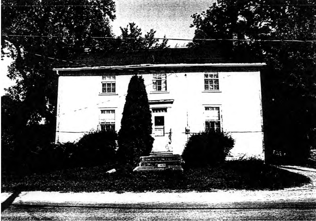
The simple three-bay symmetrical arrangement of the former May Hotel (or Letty House) is a characteristic feature of many buildings in Churchville
