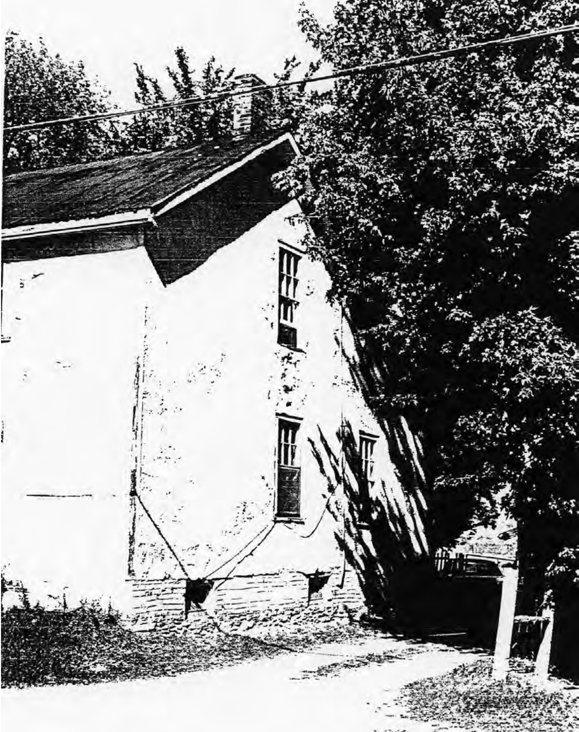
Stucco is a traditional exterior cladding and usually comprises a rendering of lime or lime and cement mortar placed on lath
