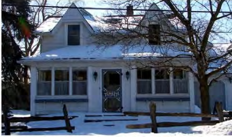
There are a number of enclosed porches in the district.
