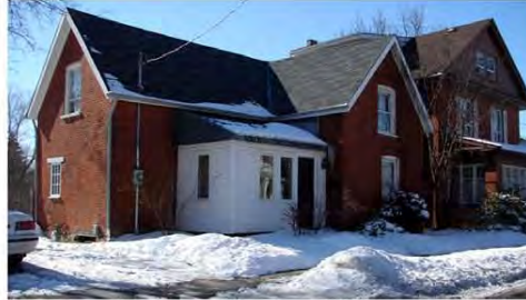
Unsympathetic vestibule addition.
