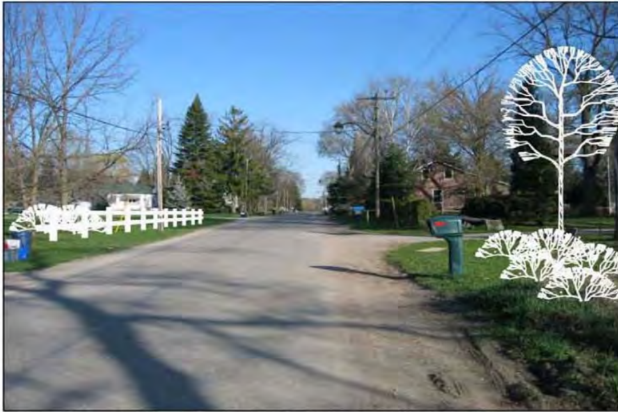
Figure 10. The rural road cross section consists of highly textured pavement (tar and chip) gravel shoulders and turf boulevards. Fencing or shrub borders may be added to define the edge of the front yard.
