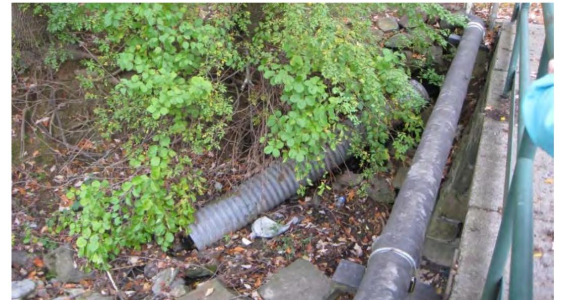
Erosion causing failure of a stormwater outfall
