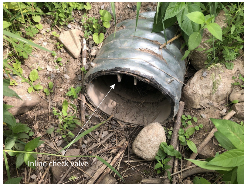
Photo 2-22: 450mm dia. CSP culvert (OF_2870) located at Segment 3 (east of bridge)
