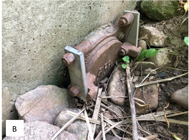
Photo 2-6: (a) Flap gate at northwest corner of floodwall segment (OF_3983) (b) Flap gate at southeast corner of floodwall with partial blockage (OF_3984)
