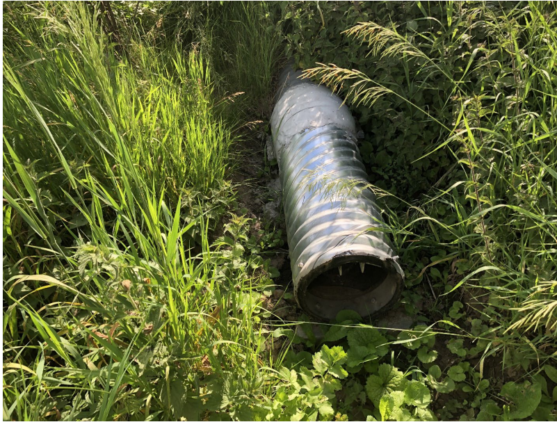
Photo 2-3: 450mm dia. CSP culvert located at Segment 1 (OF_3982)
