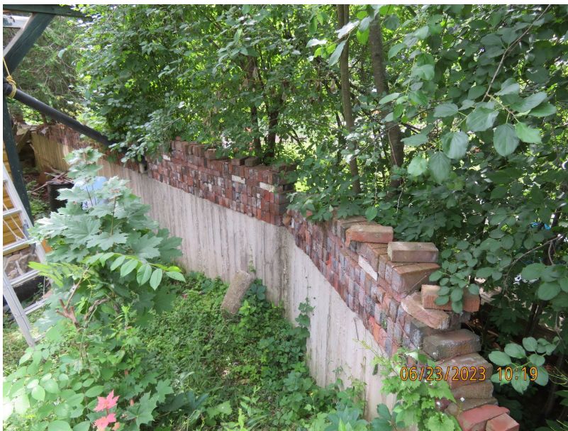
Photo 2-16: Floodwall at east of the bridge behind 11 Church Street (dry side)
