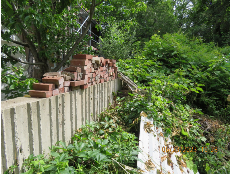
Photo 2-17: Floodwall at east of the bridge behind 11 Church Street (wet side)
