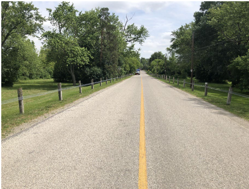
Photo 2-27: Crest of dyke along Martins Blvd (looking east)
