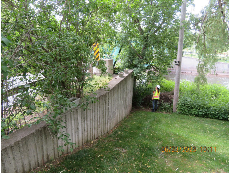
Photo 2-15: Floodwall at west side of the bridge on Churchville Road
