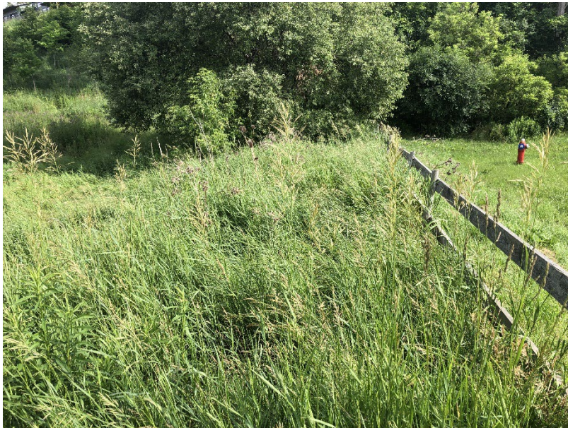
Photo 2-2: Crest and wet side slope of Segment 1, looking north
