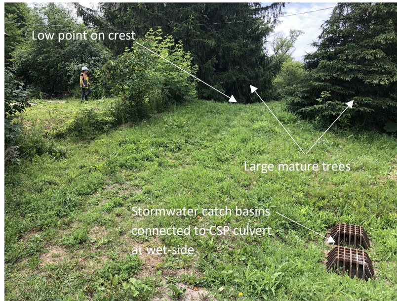
Photo 2-21: Dry side slope of berm east of bridge, looking south
