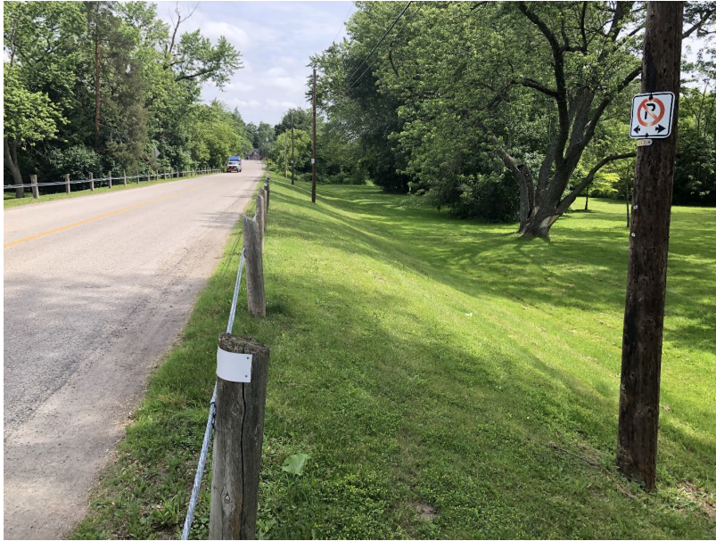
Photo 2-28: Wet side slope of Segment 5 (looking east)
