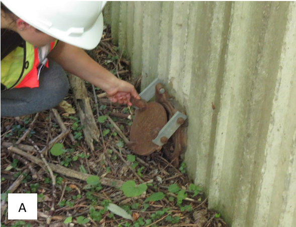
Photo 2-6: (a) Flap gate at northwest corner of floodwall segment (OF_3983) (b) Flap gate at southeast corner of floodwall with partial blockage (OF_3984)
