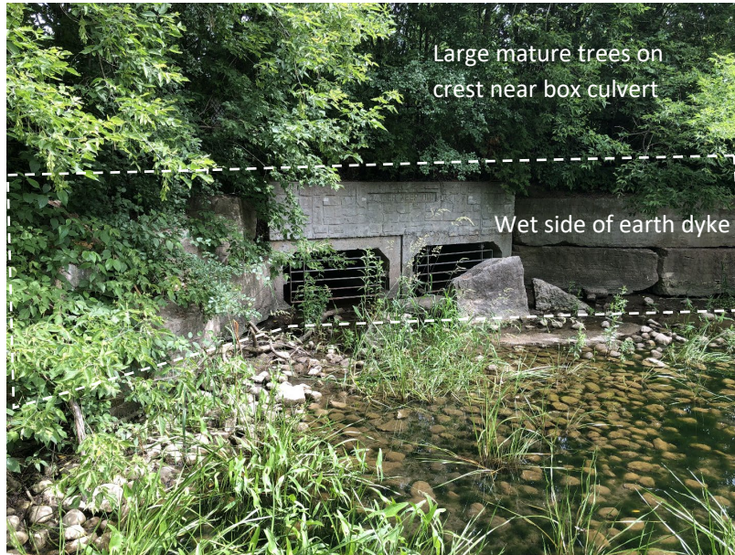
Photo 2-25: Stormwater box culvert outlet (OF_3977 and OF_3978)
