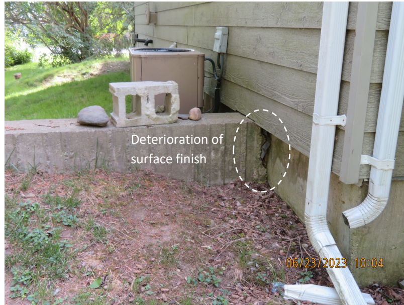
Photo 2-13: Floodwall tied into structural foundation of building at 7742 Churchville Road
