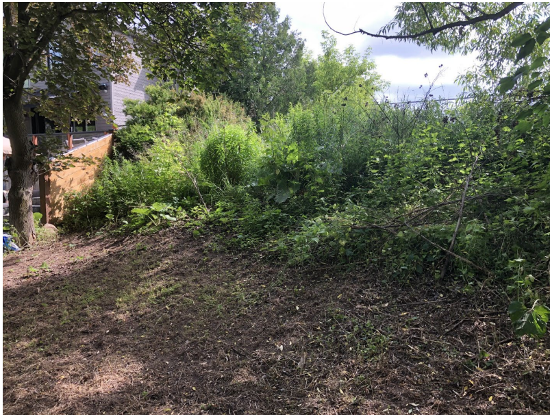
Photo 2-19: Wet side slope of dyke flanking south side of 7764 Churchville Road (looking north)
