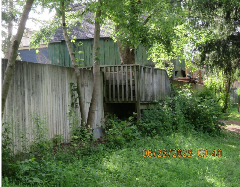
Photo 2-8: Wooden supports for the stairs anchored into the concrete floodwall
