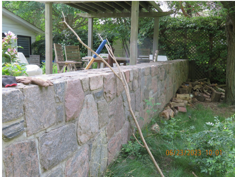
Photo 2-11: Floodwall section with stone cladding surface finish
