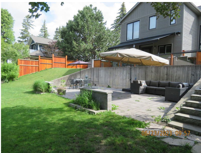
Photo 2-9: Floodwall behind 7764 Churchville Road
