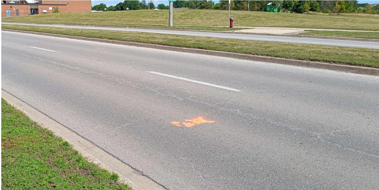
Photo 3: William Parkway, Section 1 - WB, Looking East - Location of BH P10 slight to moderate transverse cracking, moderate wheel track cracking and alligator cracking slight wheel track rutting and slight meander cracking
