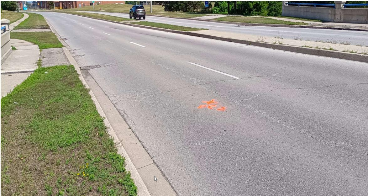
Photo 4: William Parkway, Section 1 - WB, Looking East - Location of BH EC2 slight to moderate transverse cracking, slight wheel track rutting, slight to moderate meander and midline cracking;
