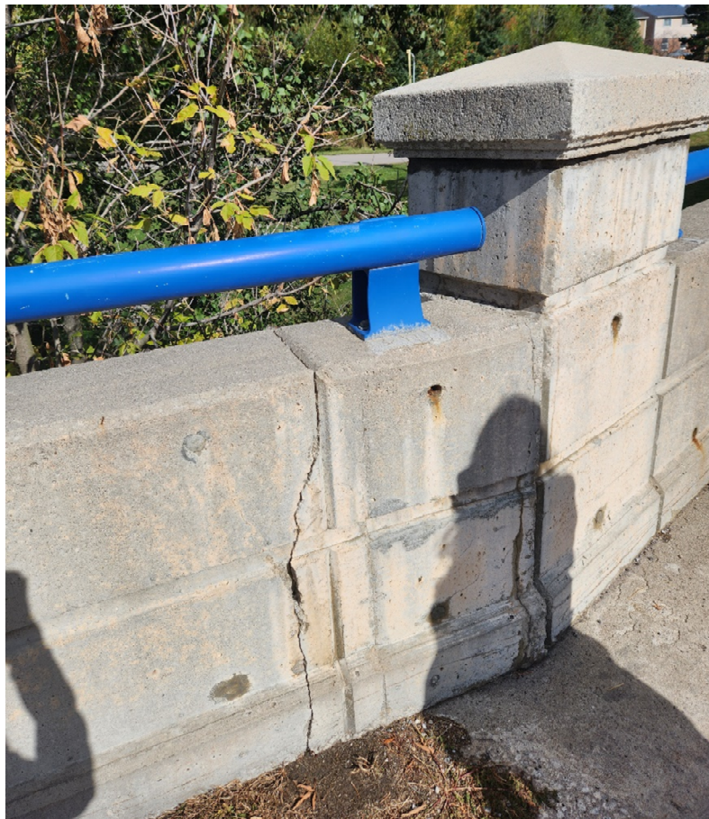
PHOTOGRAPH 20 NORTH BARRIER WALL WITH VERTICAL MEDIUM CRACKS
