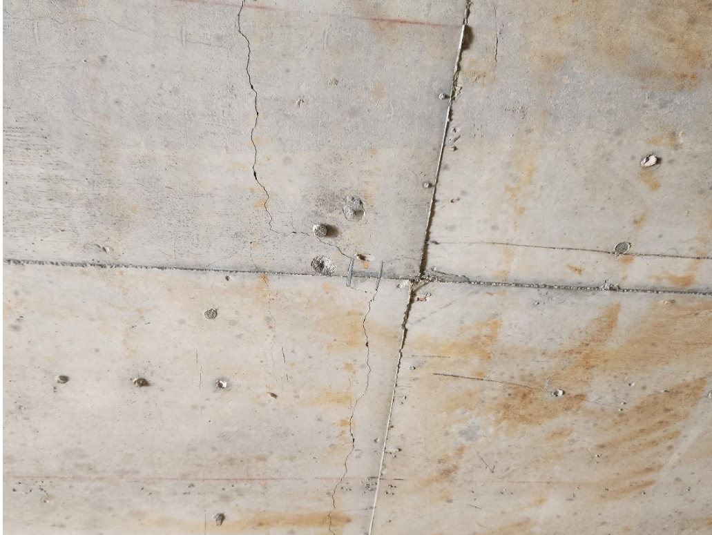
PHOTOGRAPH 23 SMALL CRACKS ON SOFFIT
