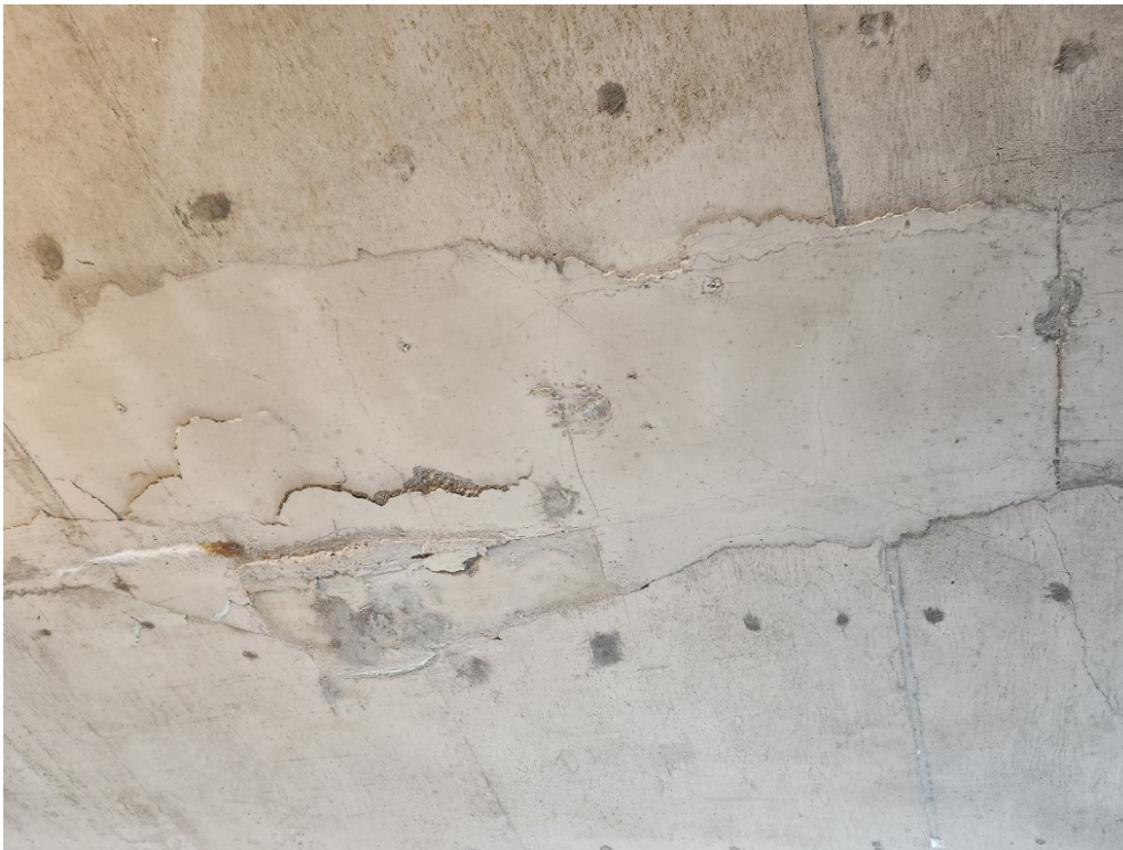
PHOTOGRAPH 22 DELAMINATION AND SPALL ON SOFFIT
