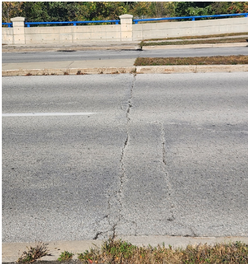
PHOTOGRAPH 2 DECK TOP LOOKING NORTH, TRANSVERSE CRACK
