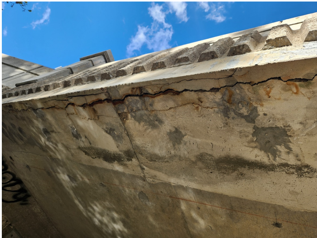
PHOTOGRAPH 12 WIDE CRACKS AT SOUTH SOFFIT
