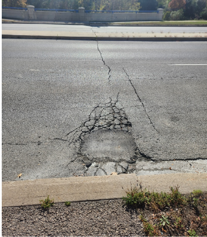
PHOTOGRAPH 3 DECK TOP LOOKING SOUTH, ALLIGATOR CRACKS
