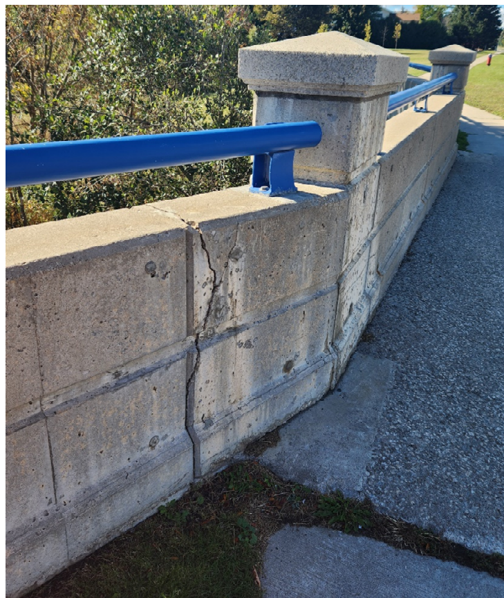
PHOTOGRAPH 18 SOUTH BARRIER WALL WITH VERTICAL WIDE CRACKS
