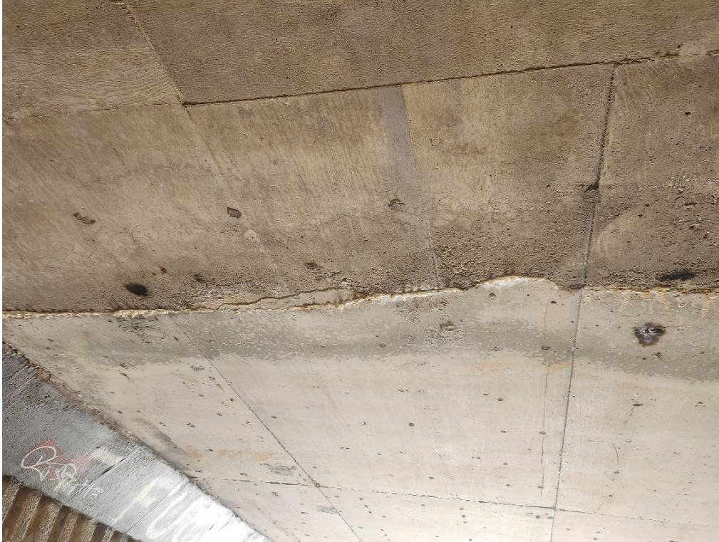
PHOTOGRAPH 21 TRANSVERSE NARROW TO MEDIUM CRACK WITH EFFLORESCENCE ON SOFFIT
