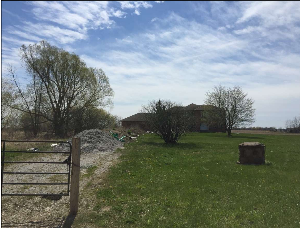
Photo 11: View of soil fill piles in front of 5253 Countryside Drive.
