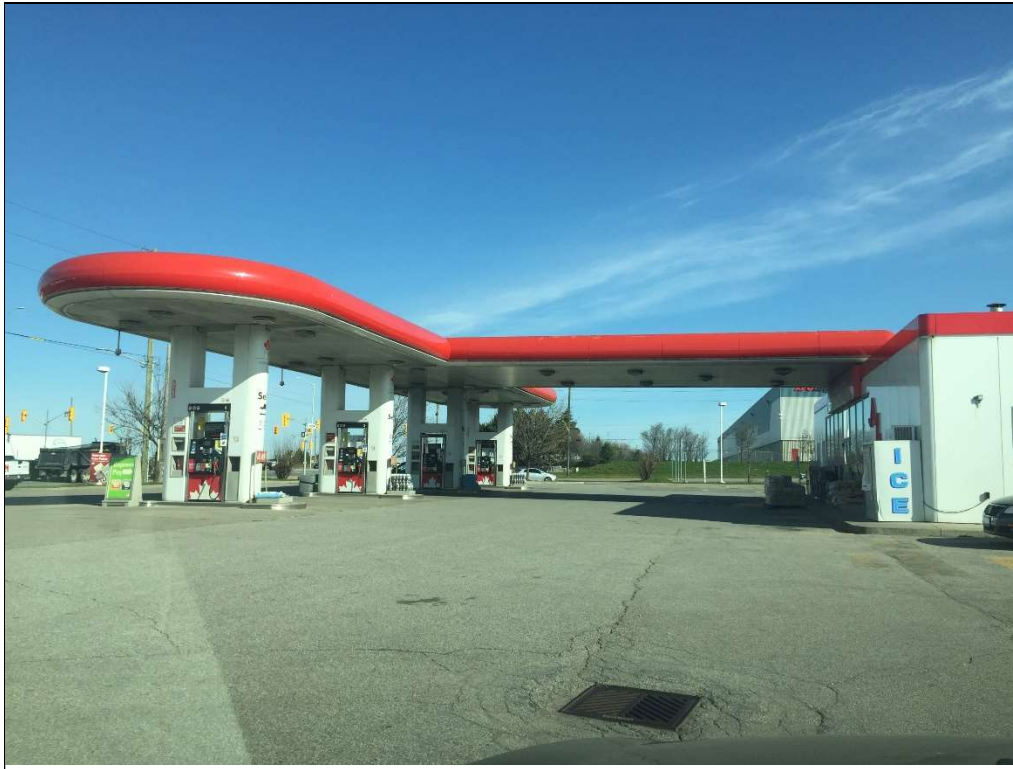
Photo 1: Gas station located at the southeast corner of Regional Road 50 and Rutherford Road.
