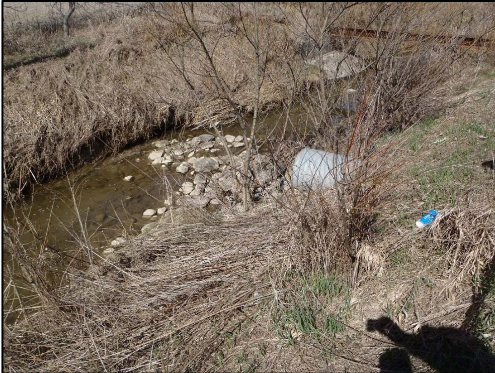
Photo 22: CTA, Reach 5. Another culvert outlets to the stream from the east. Culvert conveys flows from dry agricultural drainage ditch under the road.
