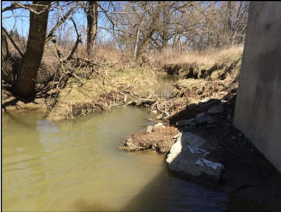
Photo 38: Crossing CT5, ROW to 20 m upstream area. Note failing bank on south bank of stream adjacent to roadway.
