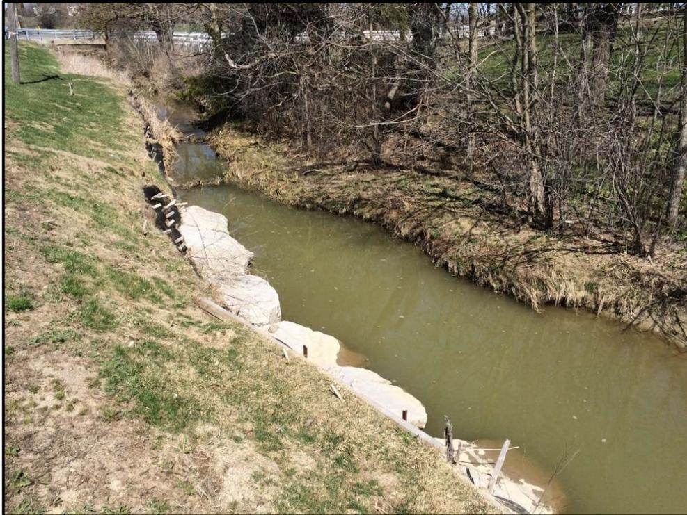
Photo 34: 50 m upstream of CT4 and 50 m downstream of CT5. Flats with staked bank treatment on west bank closest to road.
