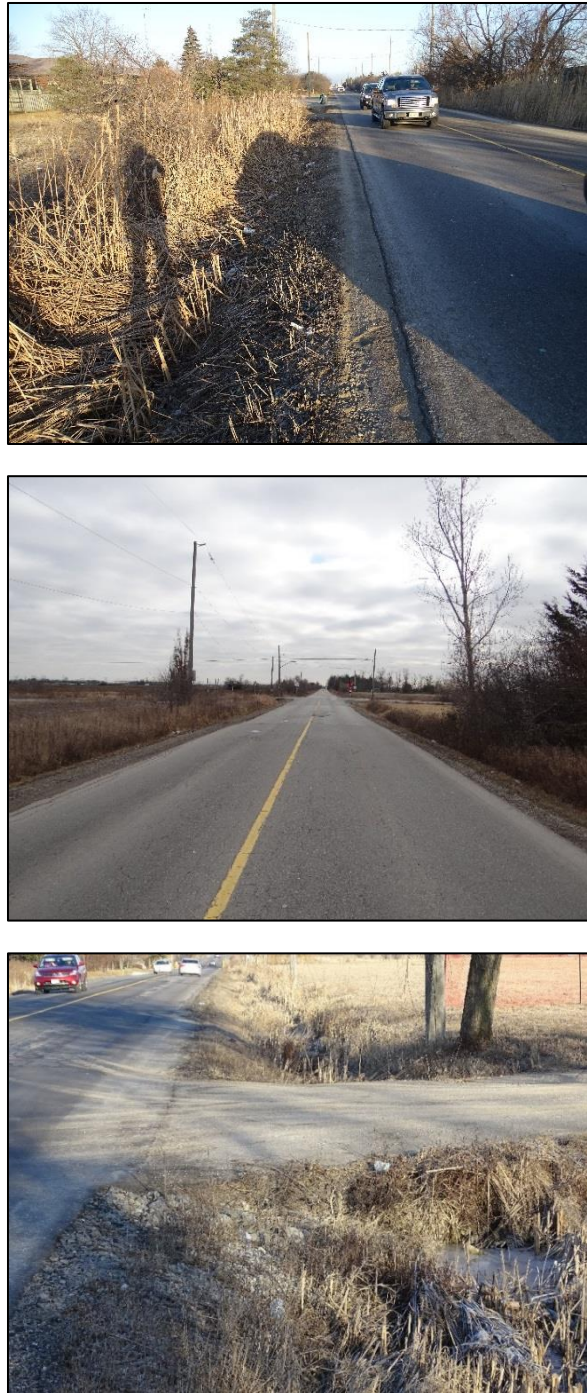
Figure 6: Narrow Shoulders along the Coleraine Drive Corridor
