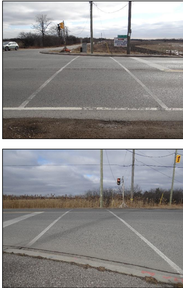
Figure 18: Offset Signal Heads (Clarkway Drive and Mayfield Road)
