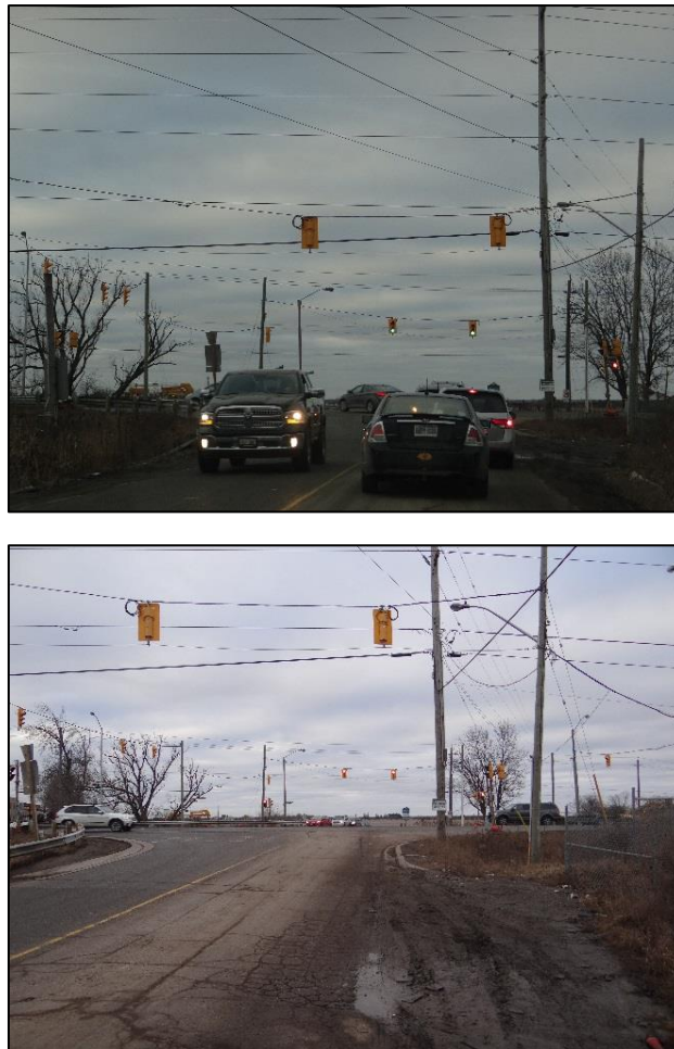
Figure 1: Elevated Intersection (Coleraine Drive and Region Road 50)
