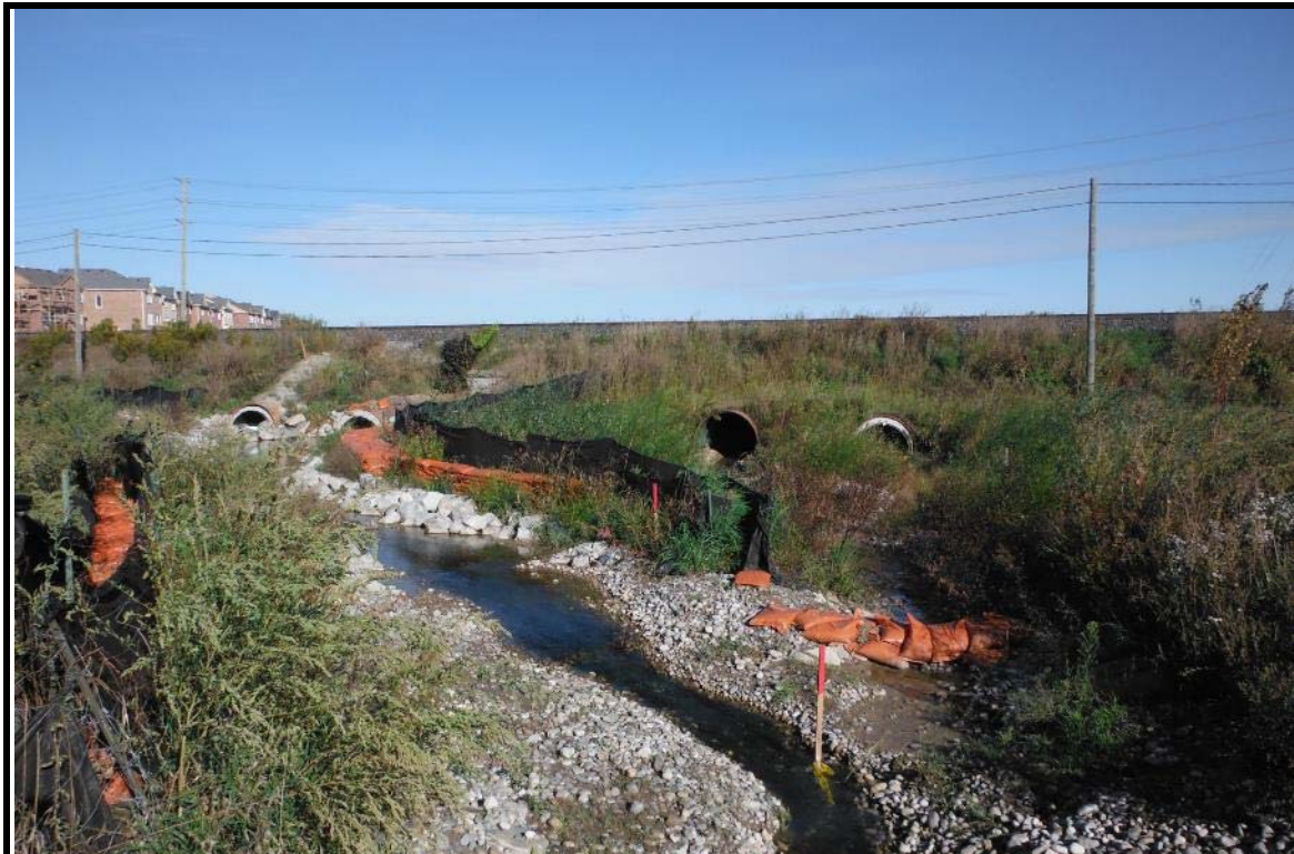
CREEK NAME: Huttonville Creek - Reach 2 FROM: Centre of Channel LOOKING: Upstream COMMENT: New channel alterations near rail line
