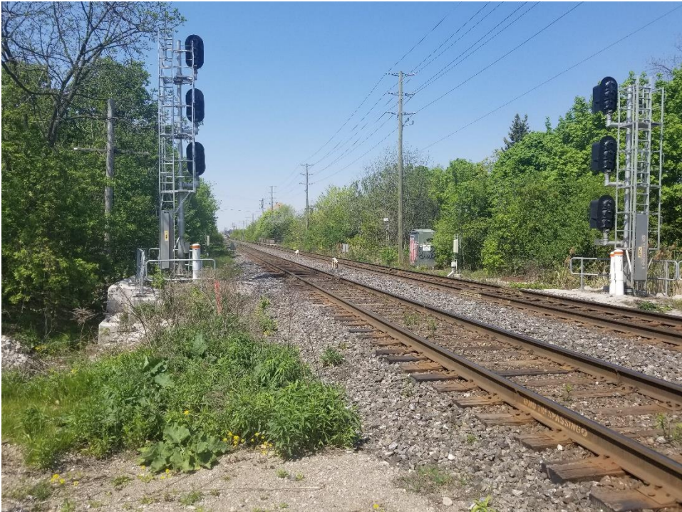
Plate 12: View of the CNR rail line at the at-grade crossing at John Street, looking west.
