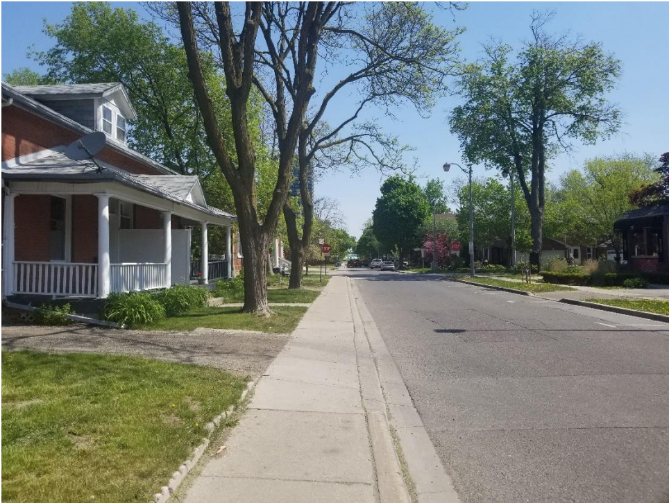
Plate 11: View of the residential properties along John Street, looking northeast.
