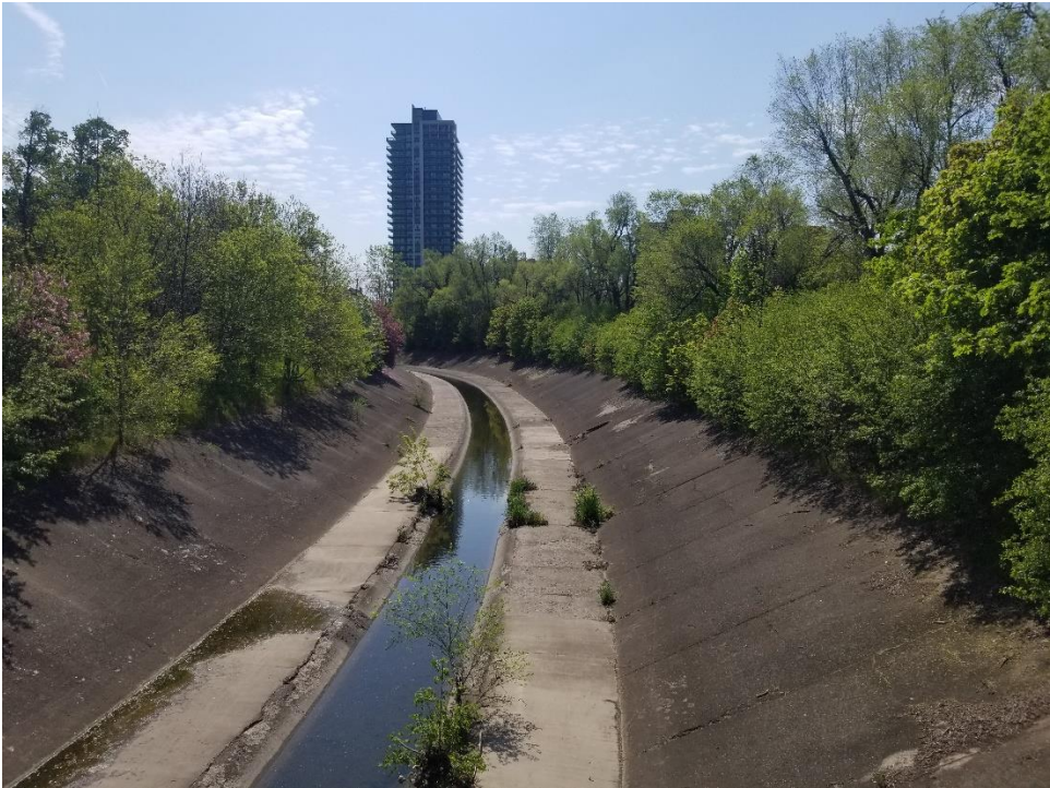
Plate 3: View of the channelized Etobicoke Creek, looking southeast from Church Street East.
