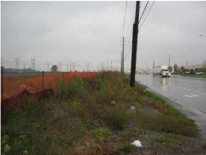
Plate 2: Looking north along west side of Goreway Dr., north of Kenview Dr., at graded lands
