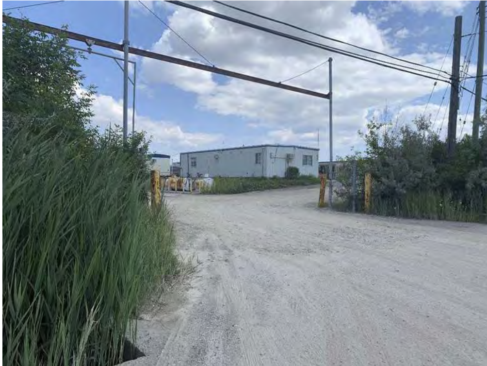
Photo 3: A view of the above ground storage tanks at 35 Rutherford Road South.
