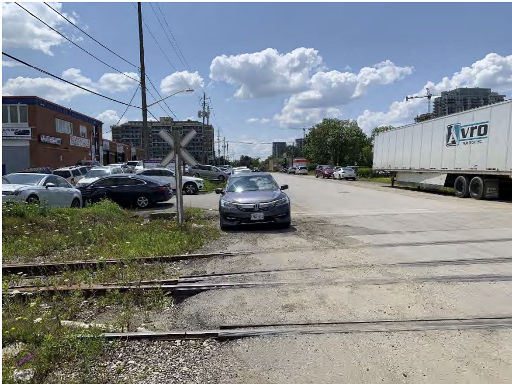
Photo 2: A view of the stains near the abandoned railway siding between 69 and 73 Eastern Avenue – View to the west on Eastern Avenue.
