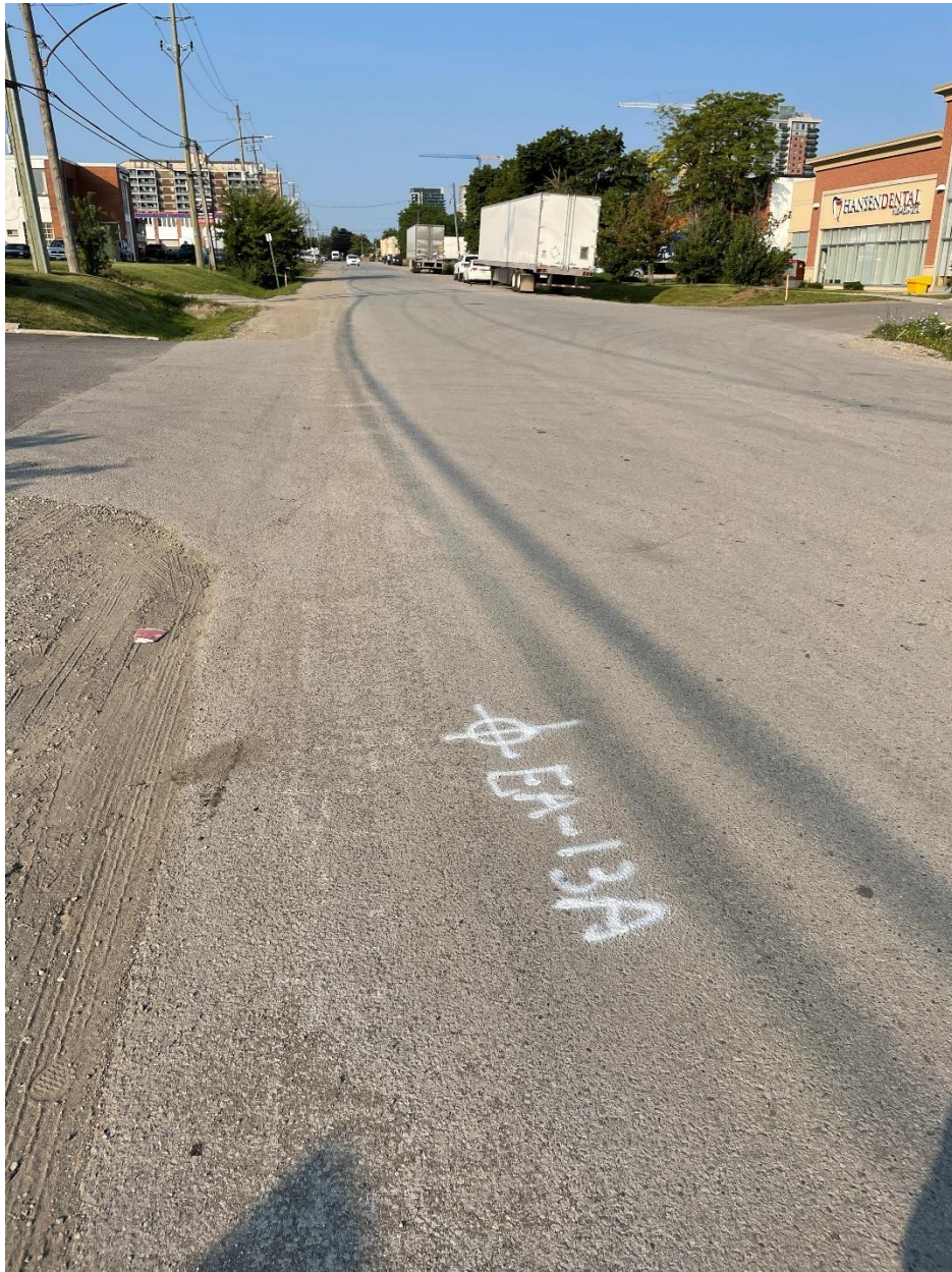
Photo 4: East end of Eastern Avenue, looking west.
