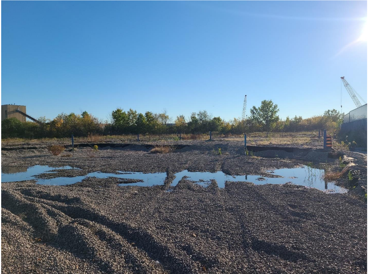
Photo 6: Property at 25 Rutherford Road, proposed Clark Extension Alignment, looking west.
