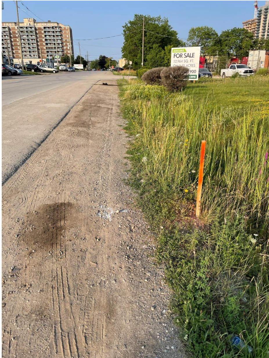
Photo 3: Eastern Avenue north shoulder and ditch, looking west.
