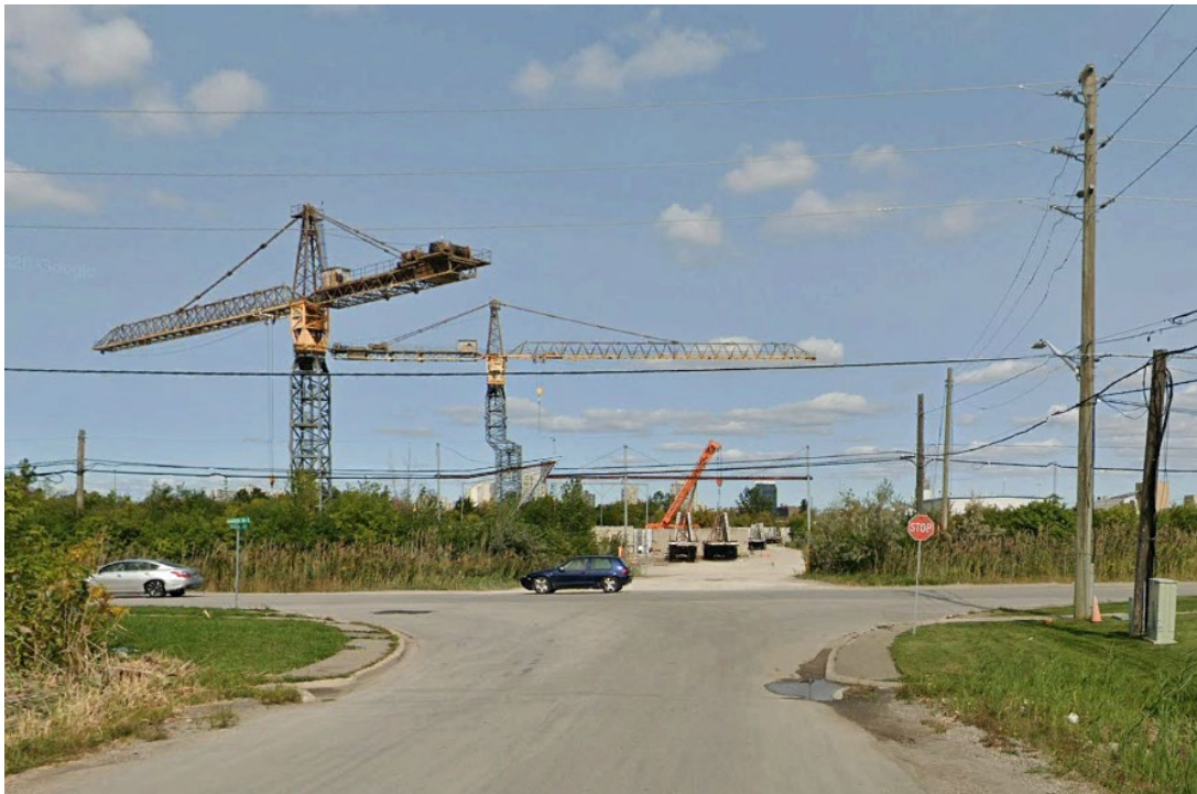
Figure 3-5: Hansen Road and Eastern Avenue (Source: Google Earth, September 2020)
