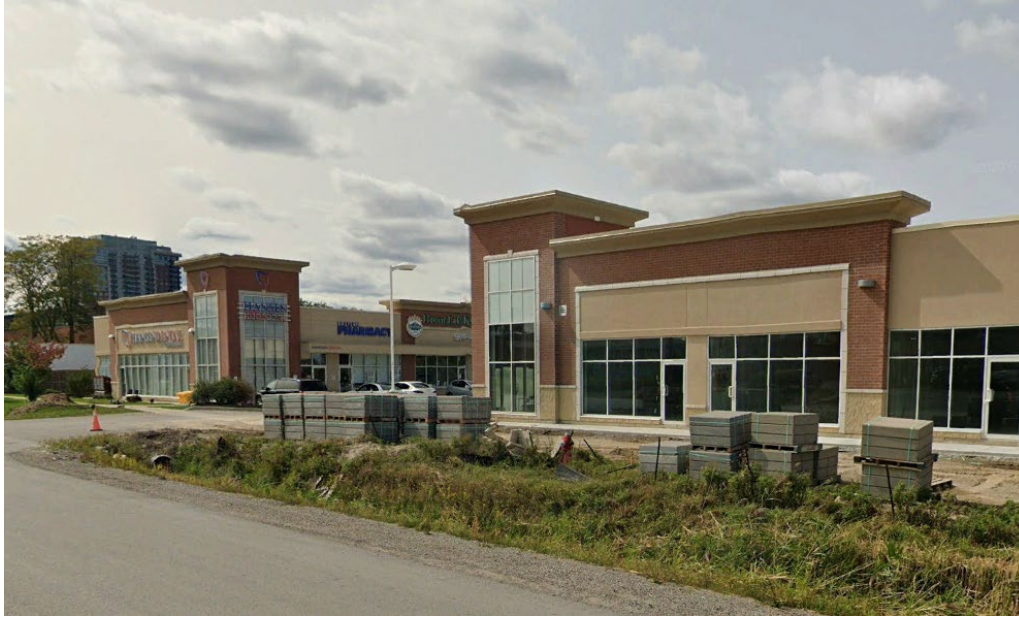
Figure 3-10: Discontinued Sidewalk at 80 Eastern Ave (Source: Google Streetview, September 2020)
