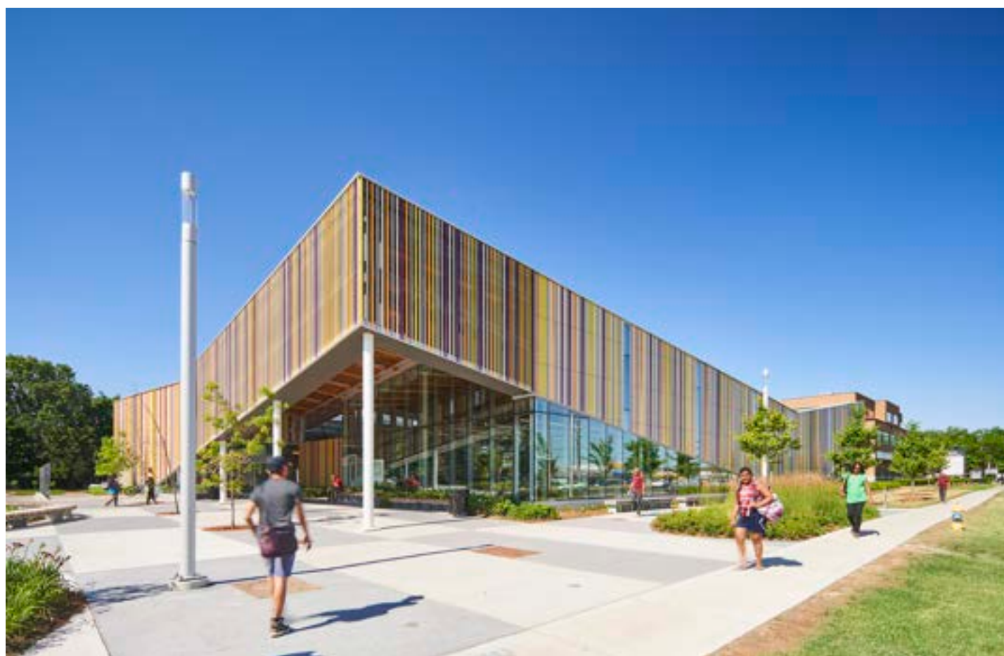
Covered Entry Plazas
