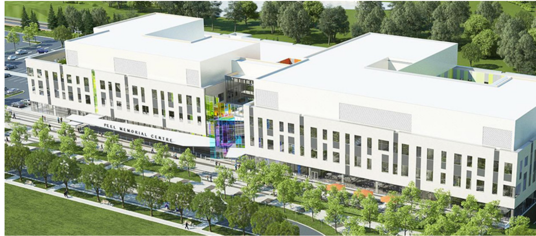
The new Peel Memorial Hospital (Brampton's second hospital)
