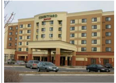
Marriott Courtyard Orion Power Centre
