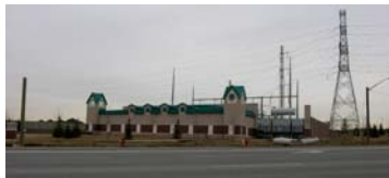
Jim Yarrow Municipal Transfer Station
