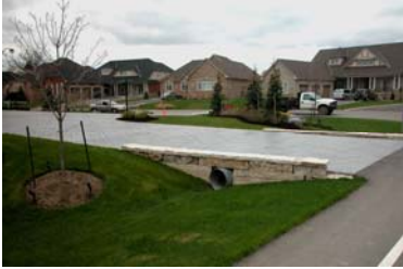
Springbrook Surface Run-off Treatment
