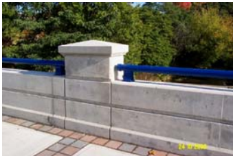
Main Street Bridge
