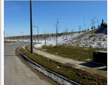
Torbram Road Noise Berm
