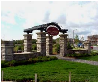
Entrance Feature, Manors of Wellington Crowne
