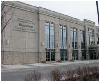
Provincial Offences Courthouse, 5 Ray Lawson Boulevard
