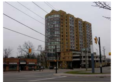
Church Street – Affordable Housing
