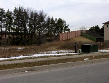
Residential Rail Noise Wall– Ravenscliffe Court
