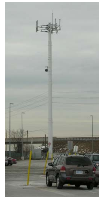
Cell Tower – Mount Pleasant GO Station
