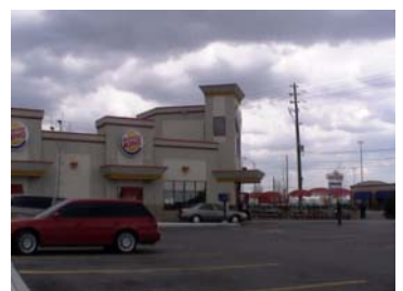
Restaurant with Drive-Thru Facility
