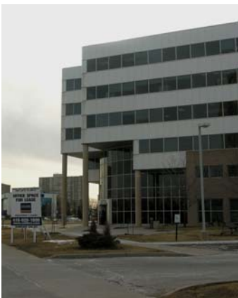
County Court Blvd – Professional Offices
