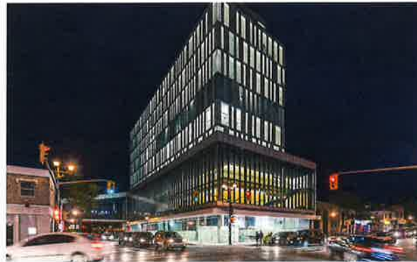
Fig 4.5.7 Downtown Brampton Street Wall
