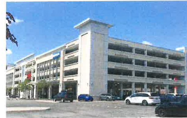
Fig 4.5.6 Aboveground Parking Garage, Bramalea City Centre
