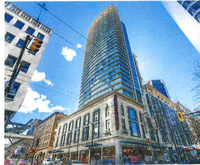
Fig 4.3.3. The Hudson, Stantec Architecture Ltd, Vancouver
