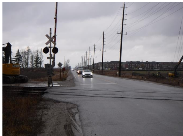
Plate 6: Railway crossing along Mississauga Road, looking northwest.
