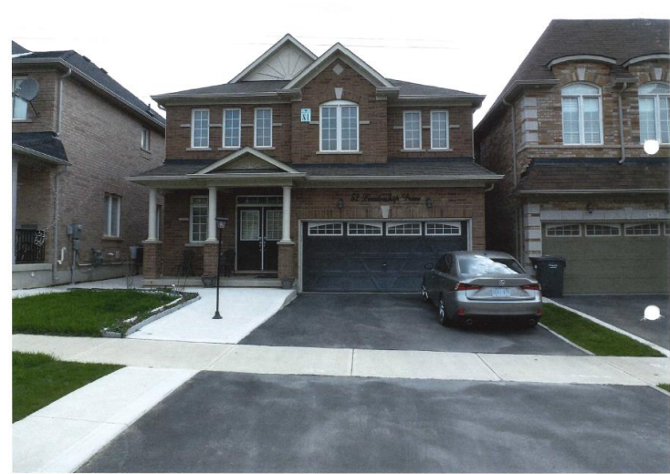
After reinstatement. The green strip does help break up impression of an expanse of asphalt/concrete.
