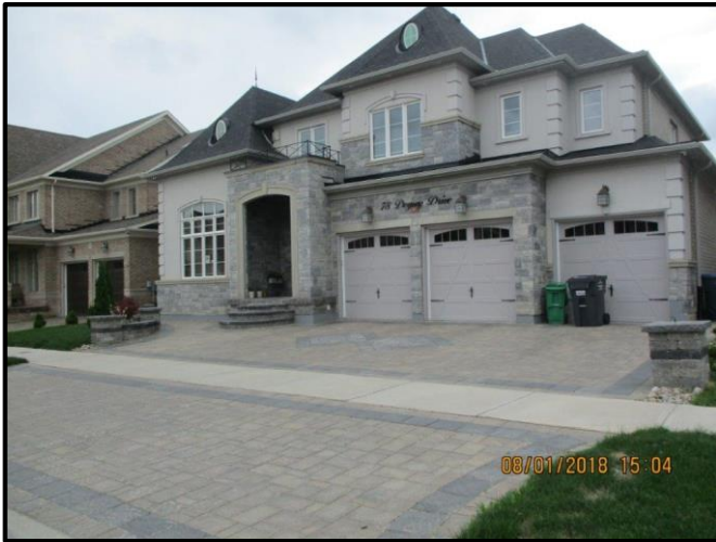
Approx. 19.8 metre lot on Degrey Drive, original driveway approximately 8.75 metres, current 10.9 metres, 0.6m permeable removed. Columns and planter may actually be in right-of-way. 9.14 metres is the maximum driveway width.
