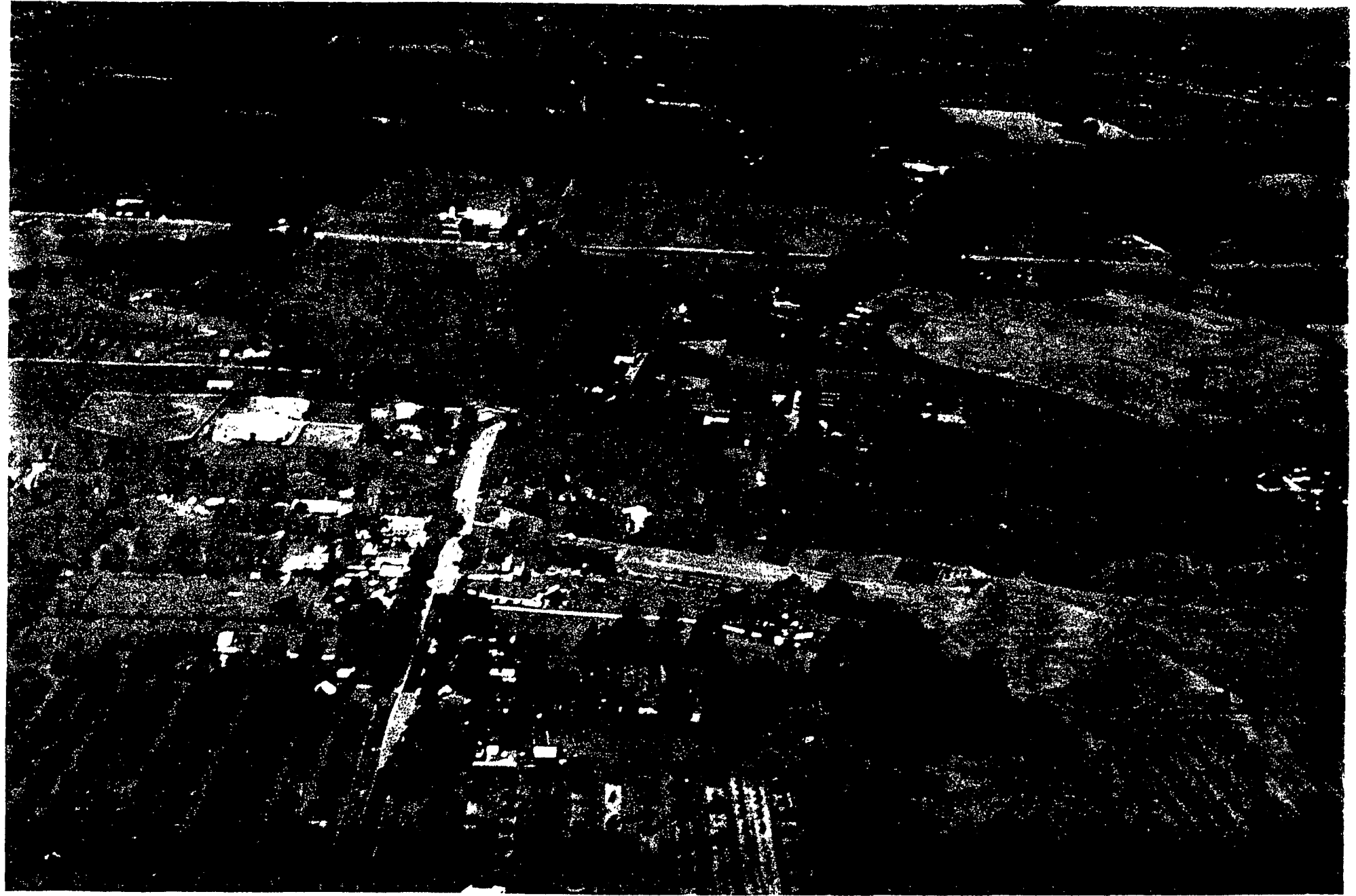
IN THE FOREGROUND IS CREDITVIEW ROAD AS IT PASSES FROM AN AGRICULTURAL SETTING (UNIT F) TO A RESIDENTIAL ONE (UNIT D) THE VILLAGE CORE IS AT THE CENTRE (UNIT A) FLANKED BY THE RIVER CORRIDOR (UNIT B) ON THE LEFT AND CHURCHVILLE ROAD (UNIT E) AND AGRICULTURAL LANDS (UNIT G) TO THE RIGHT
