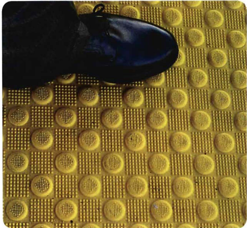
Tactile Street Material
