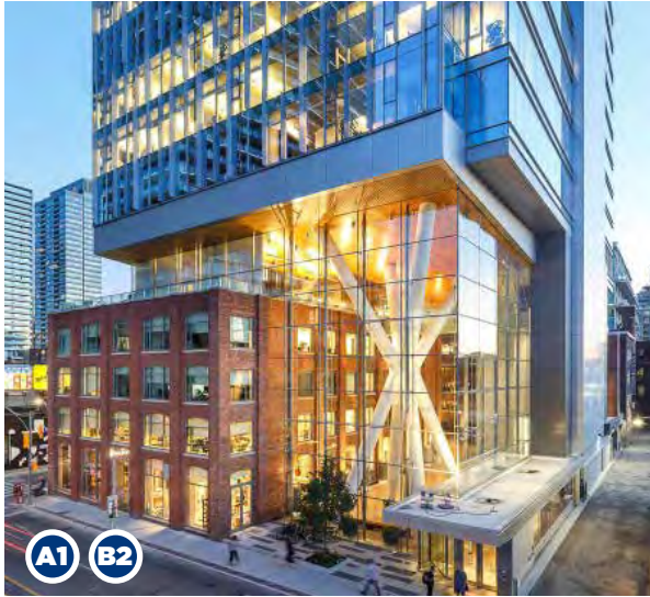
New high-rise building design to embed an existing heritage while providing steps back from the heritage - Heritage building on-site 134 Peter Street in downtown Toronto
