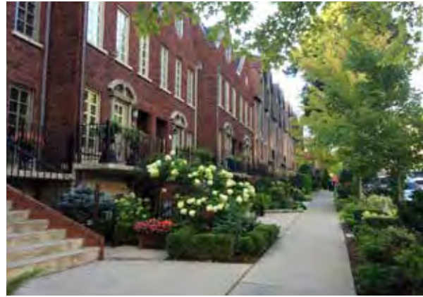
Sidewalks and Streetscaping
