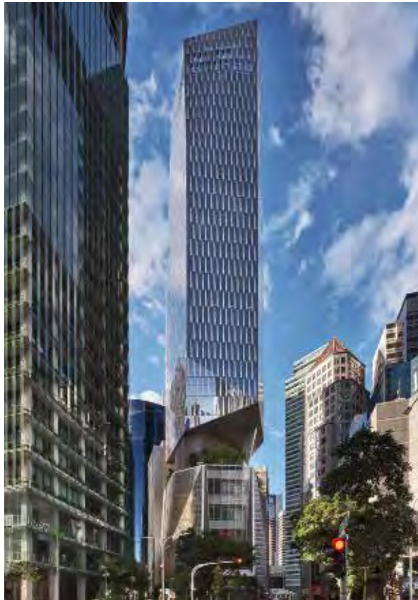
Landmark Office Building 18 Robison in Singapore
