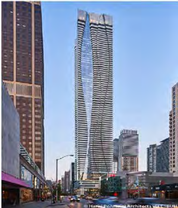
Figure 4: Minimize shadow/wind impacts through building height, massing, placement and orientation One Bloor Street in Toronto
