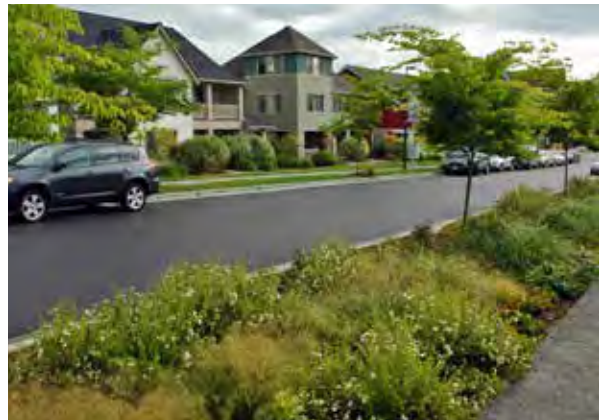
Bioswale as part of the public right-of-way
