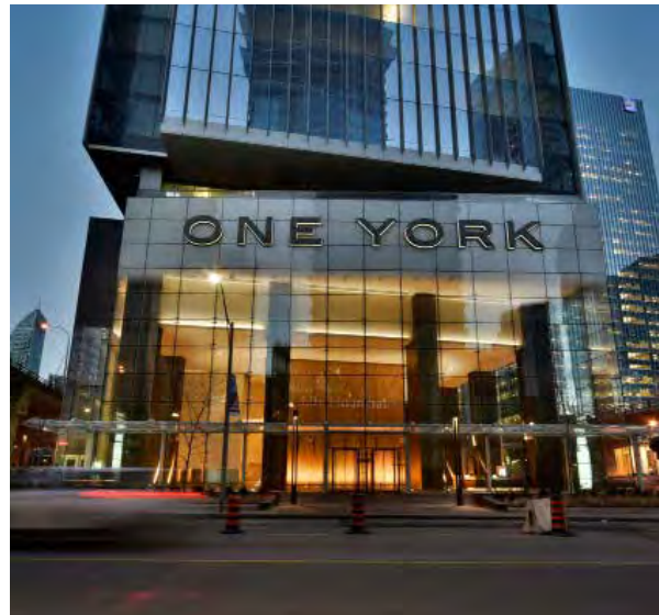
Figure 2: Cohesive elevation design between the base and the middle One York, Toronto
