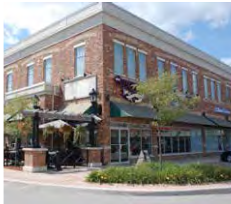
Two-storey mixed use building with retail in the ground floor
