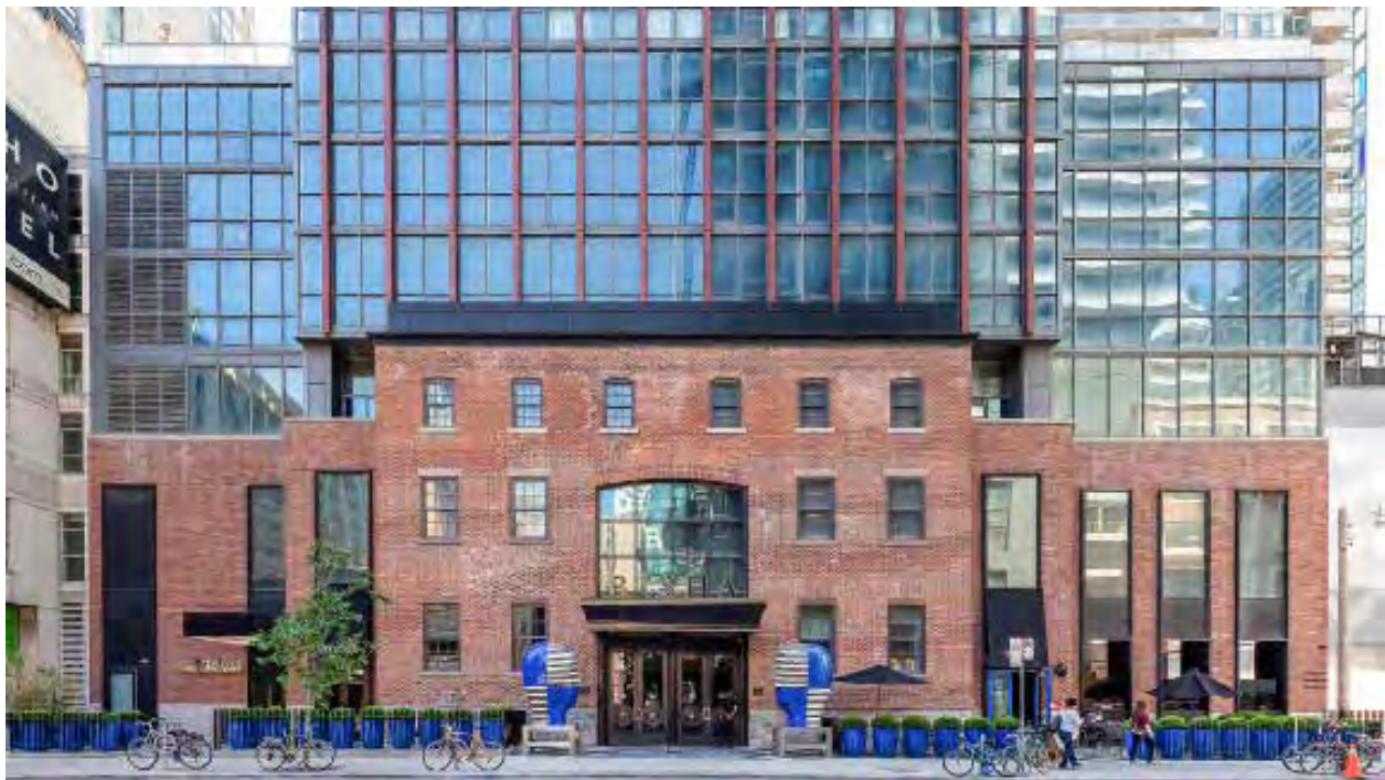
Modern high-rise building base is step back to highlight the presence of a heritage building on-site. Bisha Condo in downtown Toronto
