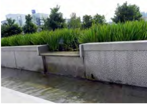
Water Treatment Features
