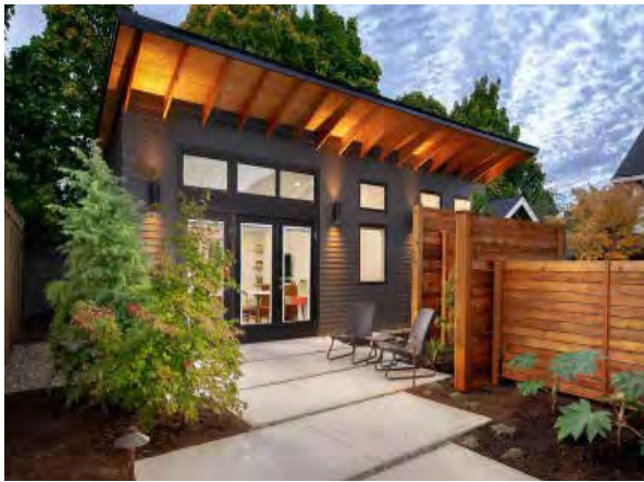
Detached additional residential dwelling
