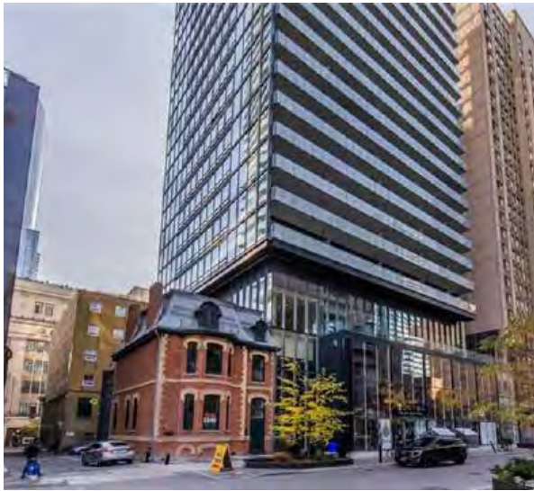
New high-rise building built adjacent to an existing heritage while keeping heritage character integration 15 Grenville Street in downtown Toronto
