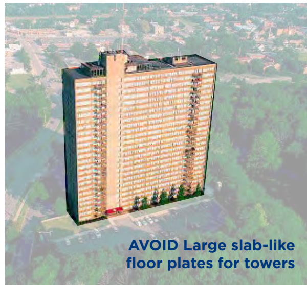
Large slab-like floor plates cast more shadow on the open spaces and streets
