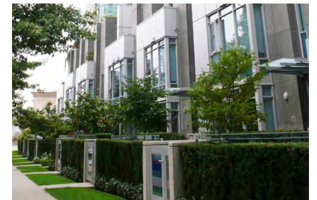
Podium townhouses (at the base of a high-rise development)
