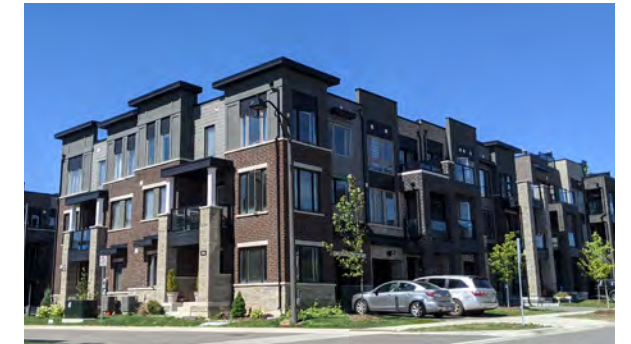
End unit at a back-to-back townhouse block
