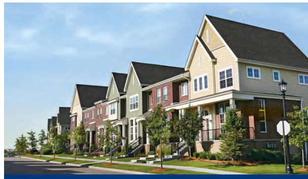
1 Create vibrant and street focused built form that frames and spatially defines the public realm.
