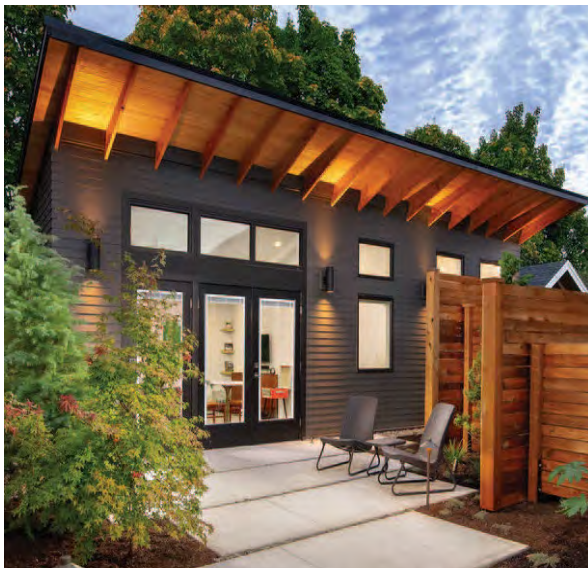
Detached additional residential dwelling
