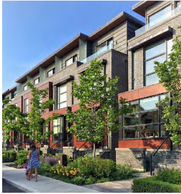
Pedestrian oriented built form
