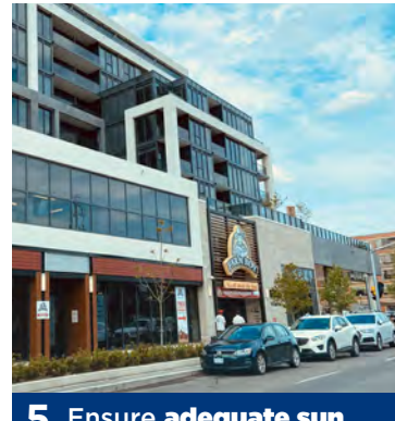
5 Ensure adequate sun penetration into the public realm and avoid adverse/extreme wind impacts.
