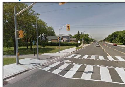
The separated crossride consists of “elephant’s feet” markings in the centre, surrounded by “zebra stripe” markings on both sides. In this configuration, cyclists are intended to use the centre part, and pedestrians the outside.
