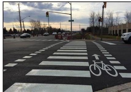
A combined crossride is comprised of “elephant’s feet” markings, with “zebra stripe” markings inside. Pedestrians are intended to make use of the central area, and cyclists to use the outer parts.
