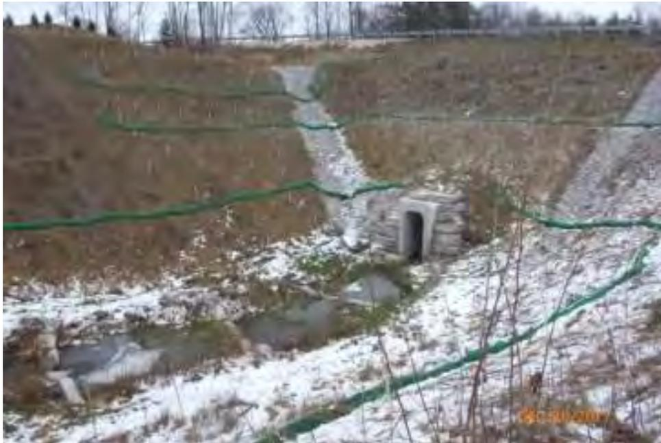
Photo 30 - Bovaird Drive West crossing CRT2-2. Stabilization at the downstream end of CRT2-2 has occurred since the original field assessment in 2011.
