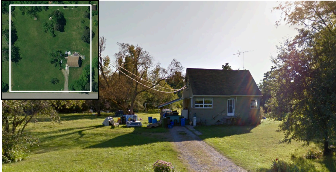
Figure 12: Example of a Dwelling with a Small Ground Floor Area
