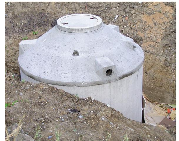
FIGURE 86 - Rainwater can be stored in cisterns.
