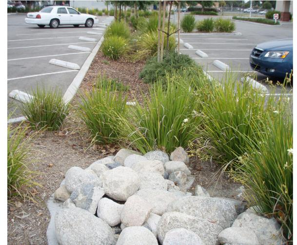
FIGURE 85 - Bioswales slow water run-off, clean and filter water, and can be integrated into street right-of-way and parking lot designs.
