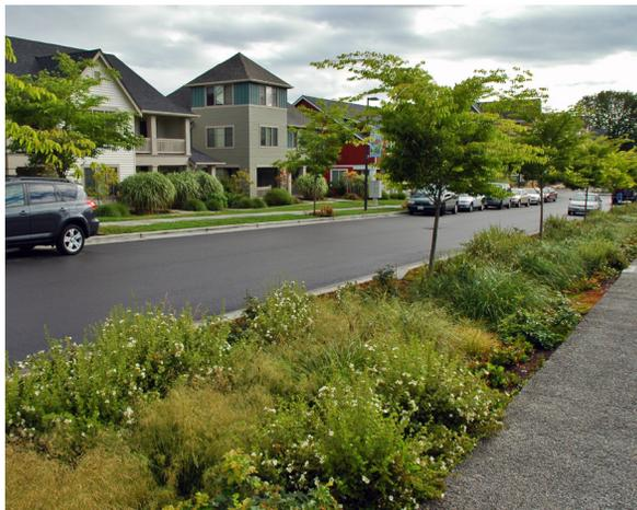
FIGURE 51 - Bioswale as part of the public right-of-way. .
