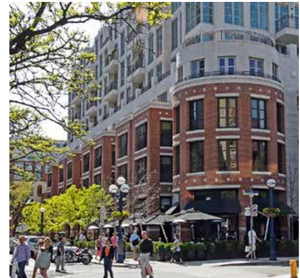
Elements such as lower cornices, canopies and material changes can provide emphasis to the ground floor.
