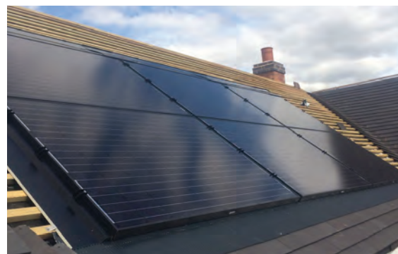
Solar panels replacing sections of roof fabric. (source: Energy Clever next generation energy solutions, Solar PV, an "in roof" solar panel system, black panels fit flush with roof tiles for more aesthetic look)
