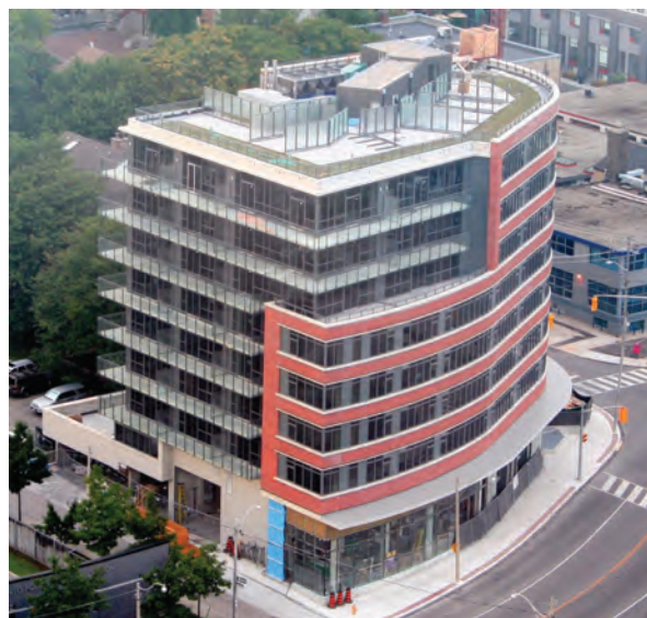
Changes in material and colour can vertically divide segments of a building to avoid monotony and reduce the impression of bulk.
