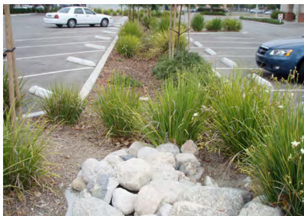
Bioswales slow water run-off, clean and filter water, and can be integrated into street right-of-way and parking lot designs.
