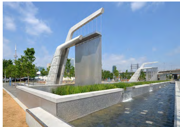
Urban Stormwater Management and Bio-filtration System
