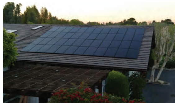
Solar panels are located within the roof line. (source: Howe Custom Home Builders, Solar Energy, 48 SunPower's Signature All Black panels)
