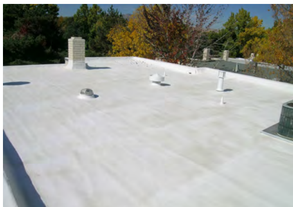
Light coloured roofs have a high solar reflectance, which reduces energy costs and reduces urban heat island effect
