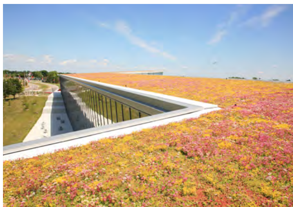
A green roof minimizes surface run-off and reduces urban heat island effect
