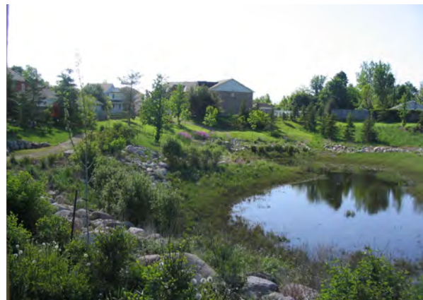
Naturalized stormwater management pond and trail system
