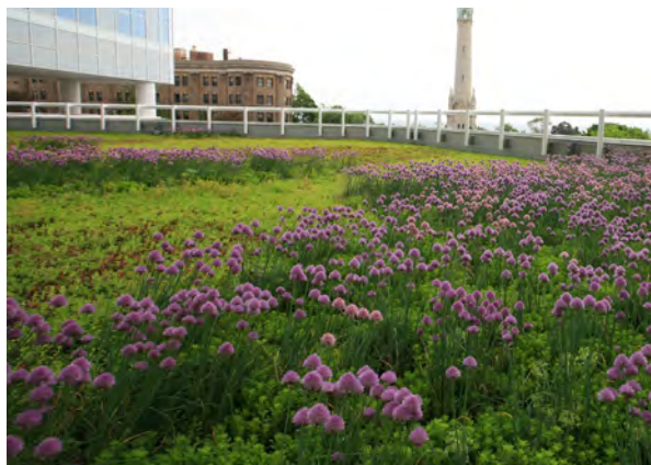
Vegetated roofs minimize surface run-off
