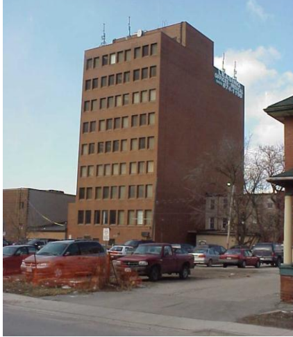
Commercial building does not integrate in context, lacks articulation and detailing
