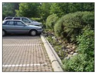
This type of LID is most applicable to employment land uses where the systems can be used to take advantage of the large impervious parking areas and where pervious landscaped areas are limited. These systems can also be used for residential driveways.
