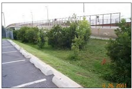
Within the Area 47 study area, filter strips may be used within the future employment lands as a pre-treatment practice for parking lot runoff before it is conveyed into adjacent biofilter or grassed swale systems. The filter strips also provide a convenient area for snow storage and treatment. Salt tolerant plantings should be used.
