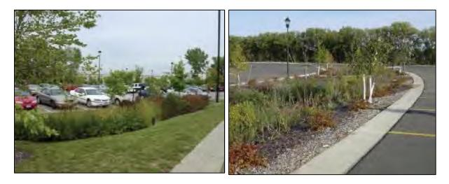
Bioretention systems are landscaped areas which capture, temporarily store, and treat stormwater runoff by passing it through engineered soil filter media. The primary component of a bioretention cell is the filter bed with a mixture of sand, soil, and organic material as filtering medium. Pre-treatment, such as a settling forebay or grass filter strip, precedes the filter bed to remove particles that would otherwise clog the filter bed. Within Area 47, this
