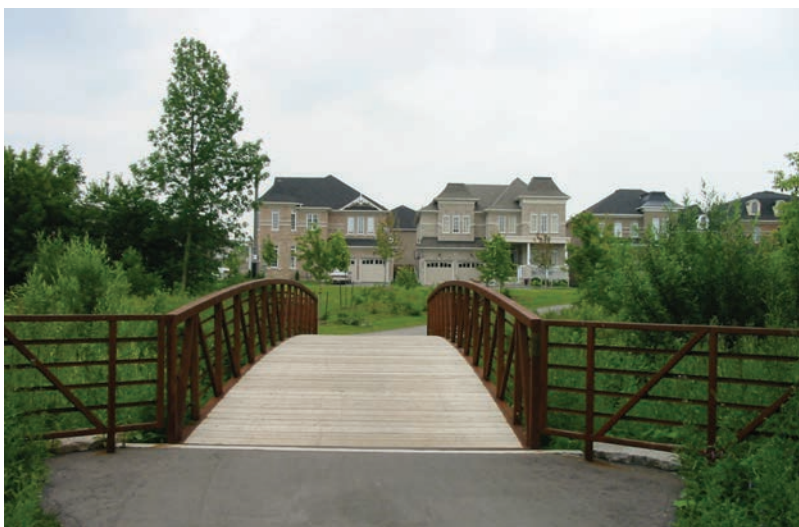
Fig. 3.3.1.1e - Image example of a pedestrian bridge crossing within the NHS with standard prefabricated steel structure and wood decking.
