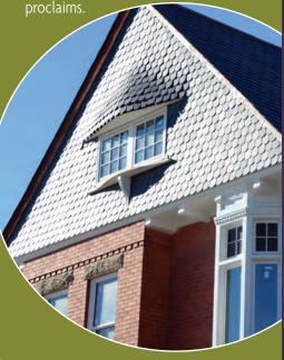
Three years later, the project is nearing completion. Work included masonry repair, the restoration and/or replication of wood features, a new slate roof, new wood sash windows, and the reproduction of the magnificent porches. The interior is also undergoing a makeover, bringing a new life to the former farmhouse
