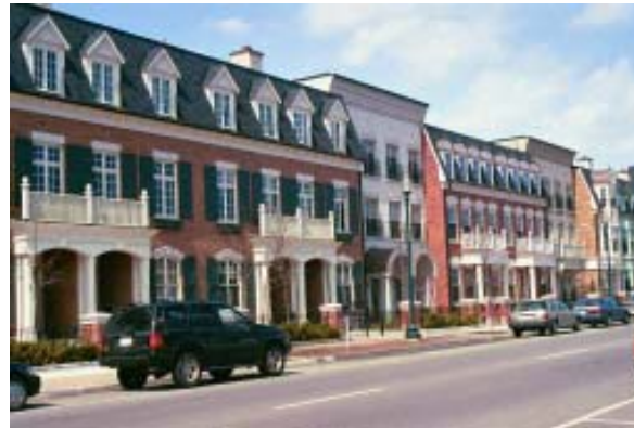
Multiple Unit Dwelling
