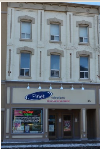
45 Main Street North current front façade
