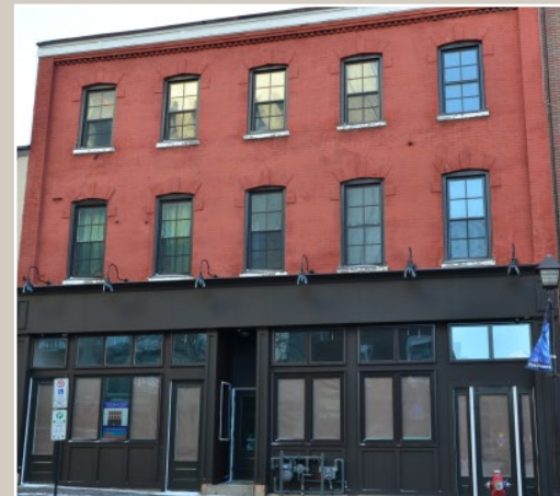
23-27 Queen Street East during façade improvement
