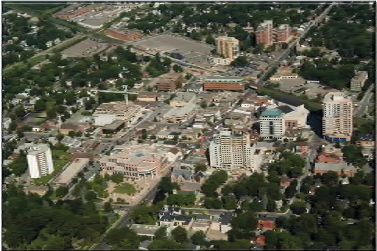
Commercial Core: View north (August 2009)
