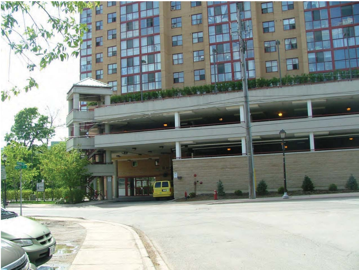
Photo 3.3 – “Wet” Floodproofing of Parking Garage, with Residences Located Above the Flood Elevation
